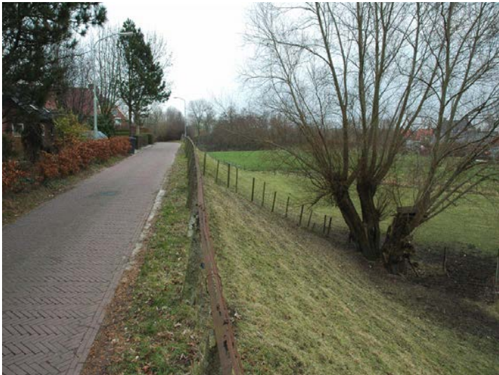
Figure 3.16: fence posts show that soil creep is a current process on the steep terp side of Wirdum after quarrying (photo: J. Meijering, Province of Groningen)
