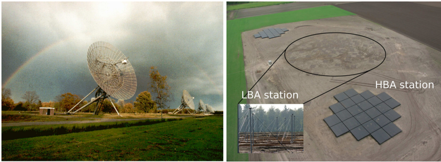
Figure 1.3: Left: Westerbork synthesis radio telescope as an example of a conventional radio interferometer (the photo's source: http://www.evbi.org/network/network.html ). Right: Core of LOFAR telescope including low and high frequency dipole fields (the photo's source: http://www.lofar.org/about-lofar/image-gallery/latest-lofar-images )
