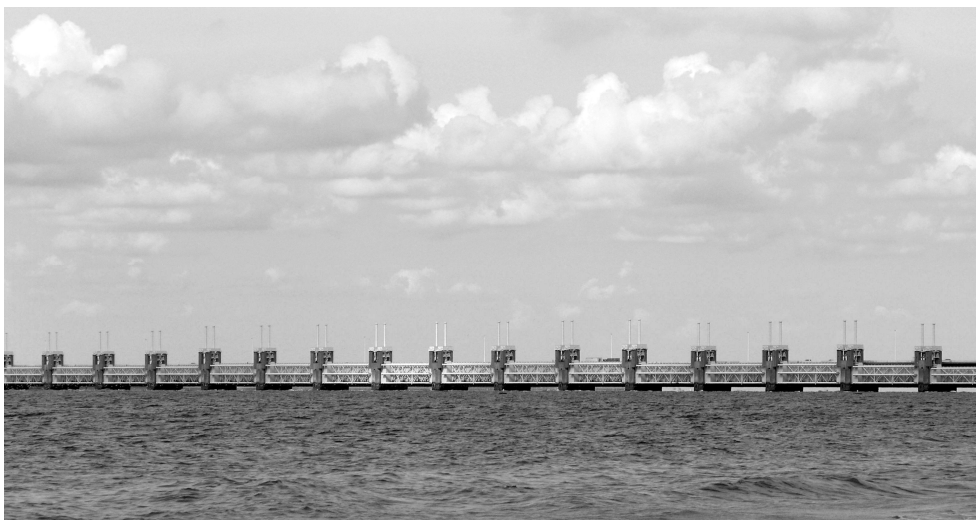
Figure B1.4.1. The Oosterschelde storm surge barrier, viewed from the North Sea.
