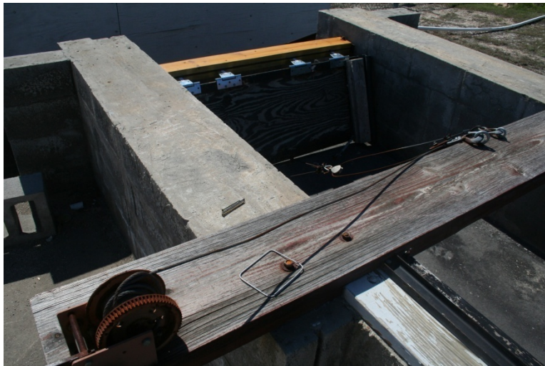
Figure 3.10 – Tailwater Gate
