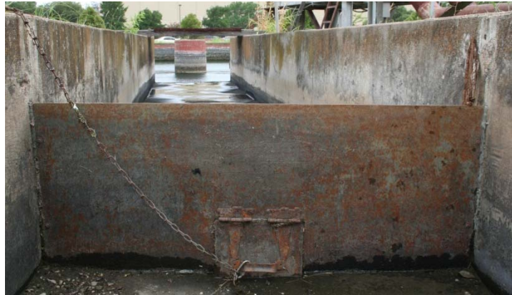
Figure 3.5 – Sharp Crested Weir
