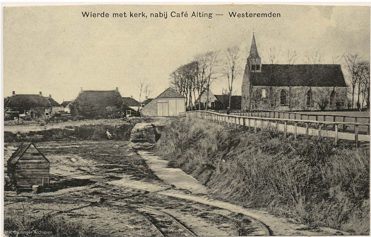
Figure 3.1: Example of quarrying a terp (Westeremden) in the early 20 th century, leaving a steep face and a pedestal-shape terp body (Picture Collectie Groninger Archieven, www.beeldbankgroningen.nl (1173-143-102))
