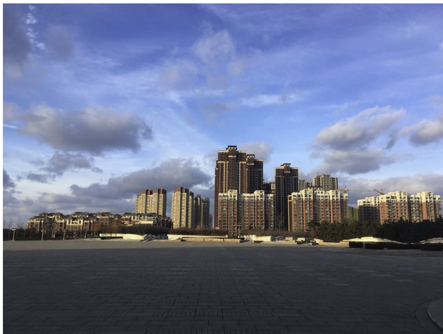
Fig. 4. The new buildings in Beizhai village (Dec 2017). Source: Chen Chen.
