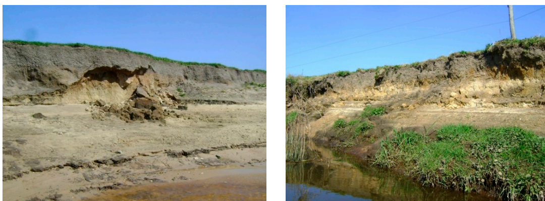
Figure 5. Examples of active bank erosion. Bend 124 (left) and bend 101 (right).
