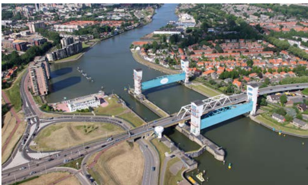
Figure 1: The Algera Complex [beeldbank.rws.nl].
