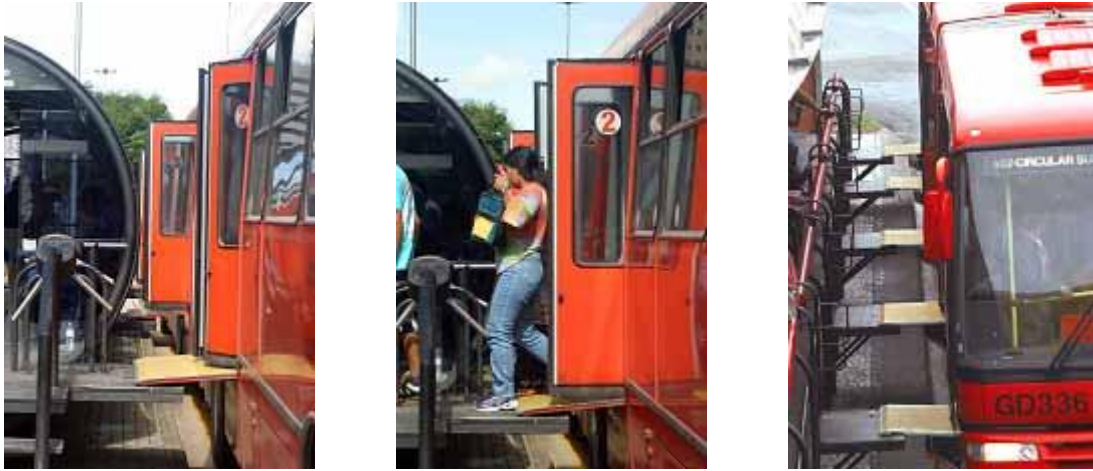
Fig. 5.4 Boarding System at Station level
