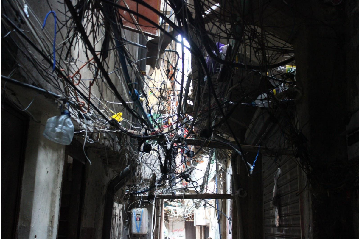
Common image of streets in Burj El Barajneh Palestinian Camp. Water pipes, electricity wires, telephone wires and internet wires are distributed by hanging over alleyways. © Nihal Halimeh, 2017
