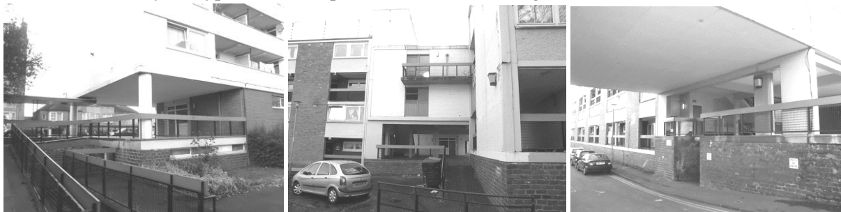
Figure 2. Claremont Court. Types of entrance and relation with the street.
