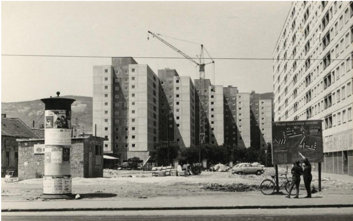
Figure 1. Construction of Óbuda Housing Estate in 1967 – prefabricated modern housing replaced the former historic urban fabric
