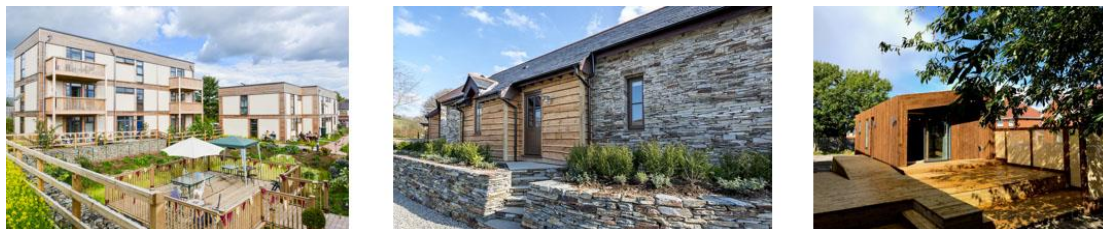
Fig 4, 5 & 6. Examples of straw bale panel constructions in 3 differing house styles; Lilac Co-housing in Leeds, Yeotown Eco-Lodges and TAM, a cosy, 'mini' home. Using naturally-grown straw as insulation means the houses are Carbon-positive and healthy. Images courtesy of ModCell.
