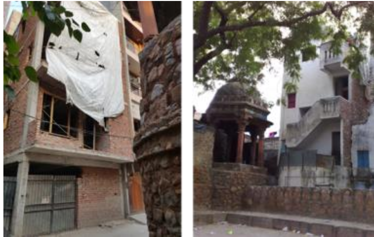
Figure 7. Construction activity and buildings adjacent to the protected “Moth ki Masjid.”
