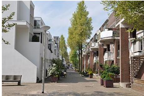
1978-82 - The Haarlemmer Houttuinen in Amsterdam, designed by Herman Hertzberger The pedestrian street, entrances and balconies are situated behind the pillars.
