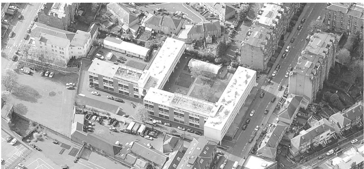
Figure 1. Claremont Court housing scheme. View of the two L-shaped volumes around the landscape courtyards
