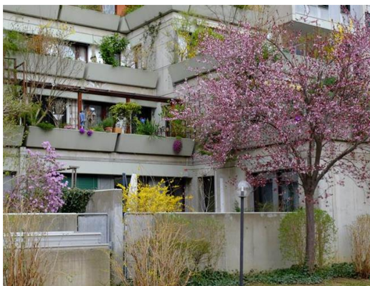
Figure 4. Renovated concrete in Terrassenhaussiedlung St. Peter, 2015
