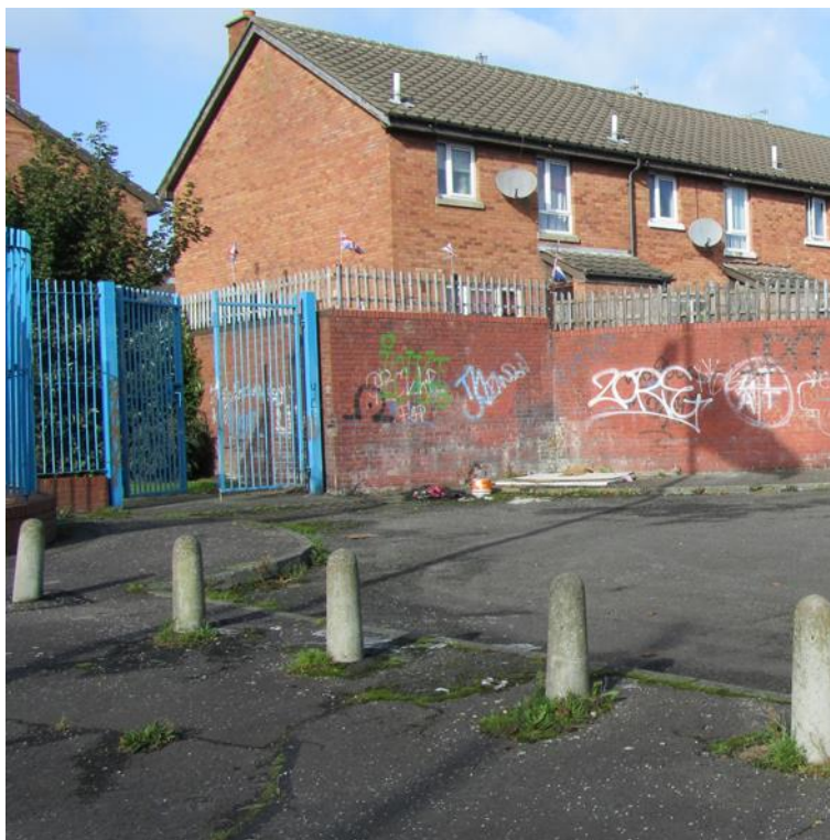
Figure 4 Bollards preventing vehicle access to the rear of walled courtyards, Cupar Way, West Belfast
