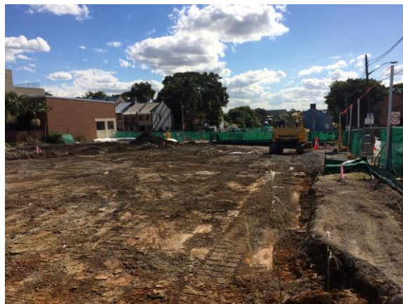
Figure 1. Demolition of homes
