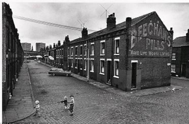
Figure 1. Terraced Housing built in the 1900's shown in the 1960's 3
