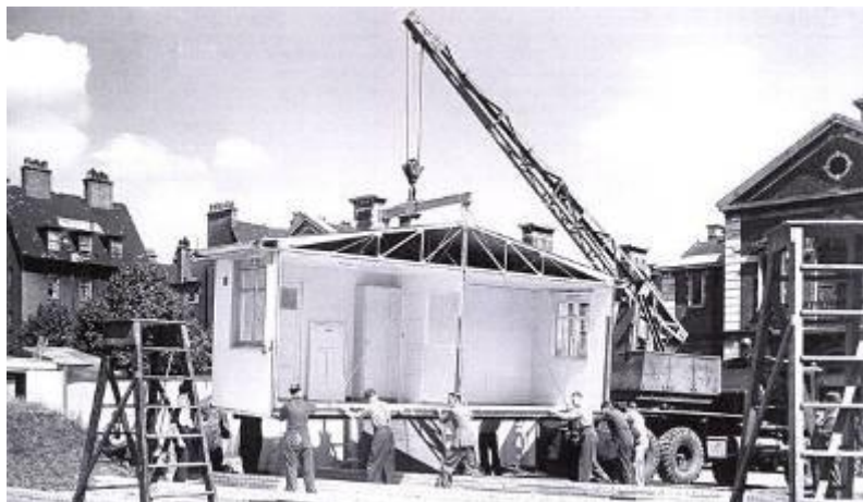
Figure 2. prefabricated house built using 'war' technology 4
