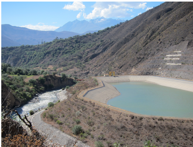
Figure 12: One of two reservoirs built just upstream of Cañon del Pato for storage; Photo by Laura Read
