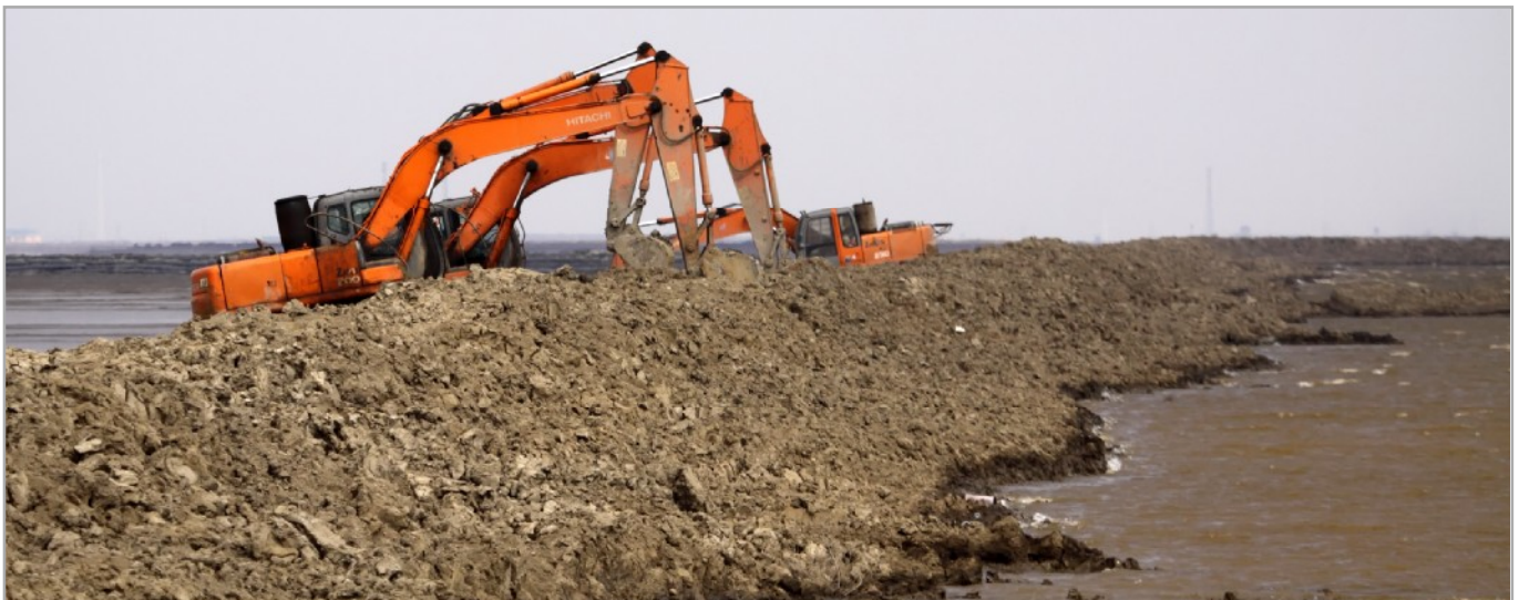
Seawall construction at Beipu April 2014 © Matt Slaymaker
