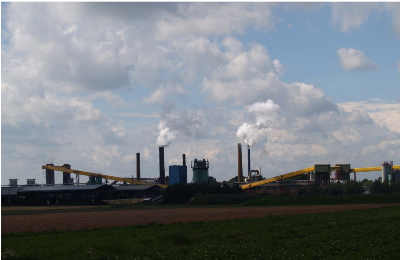
Figure 5. The Purit plant in Klazienaveen, 2000.
