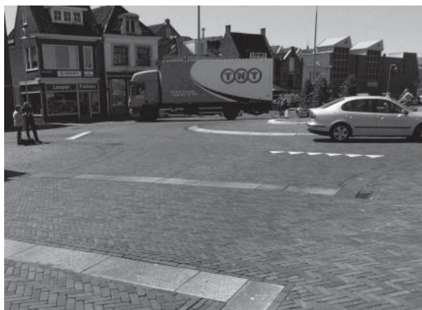
Figure 3. Sneek (Prins Hendrikkade). In the front there is a crossing suggestion, marked by grey stones amongst dark red paving.
