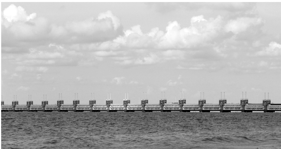
Figure B1.4.1. The Oosterschelde storm surge barrier, viewed from the North Sea.
