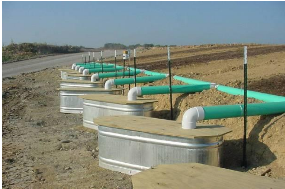
Figure 3-3 Test Plots with Runoff Collection System and Rain Gauge
