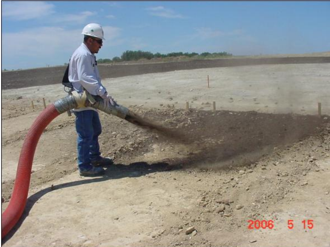
Figure 3-5 Installation of Erosion Control Compost
