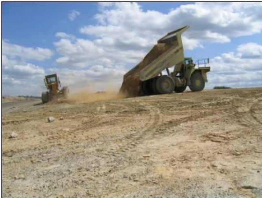
Figure 3-2 Construction of Test Plots
