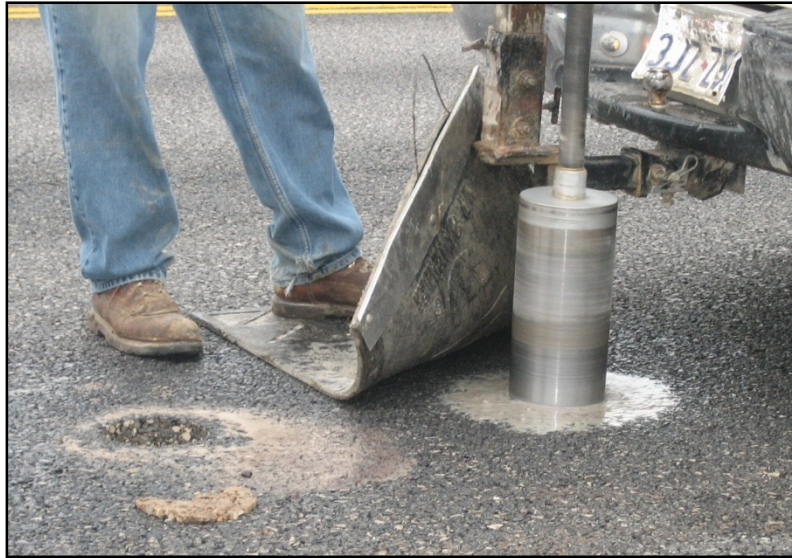
Figure 6 - Drill Press on RM 620 - March 14, 2007
