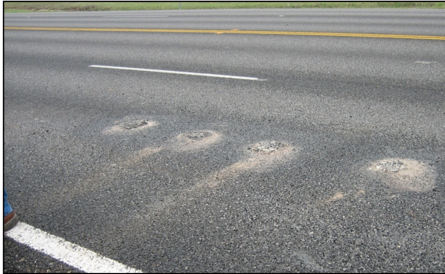
Figure 8 - Quick pavement filling holes on RM 620 - March 14, 2007
