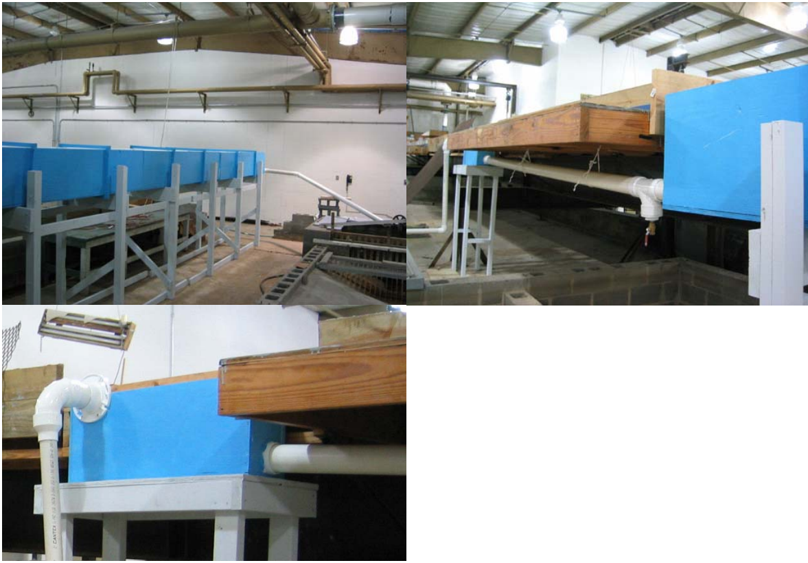
Figure 4.1. The first sedimentation basin, built in 2003, caused a lot of problems (Top-Left: Sedimentation basin set on wooden supports (view from inlet to outlet), Top-Right: mixing box, 3-inch pipe connecting mixing box and sedimentation basin, and Bottom-Left: mixing box)
