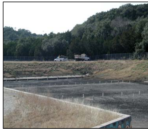
Figure 2.2 Sand Filter Basin
