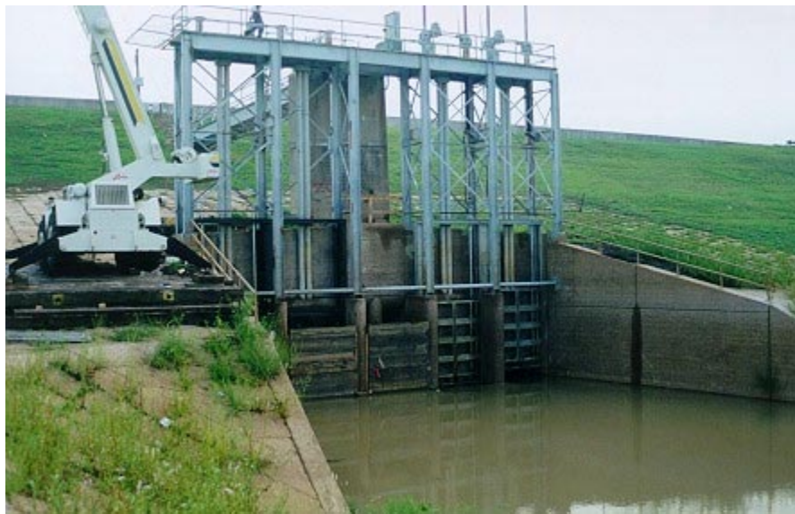
Figure 3.7: Exit point of Addicks Reservoir
