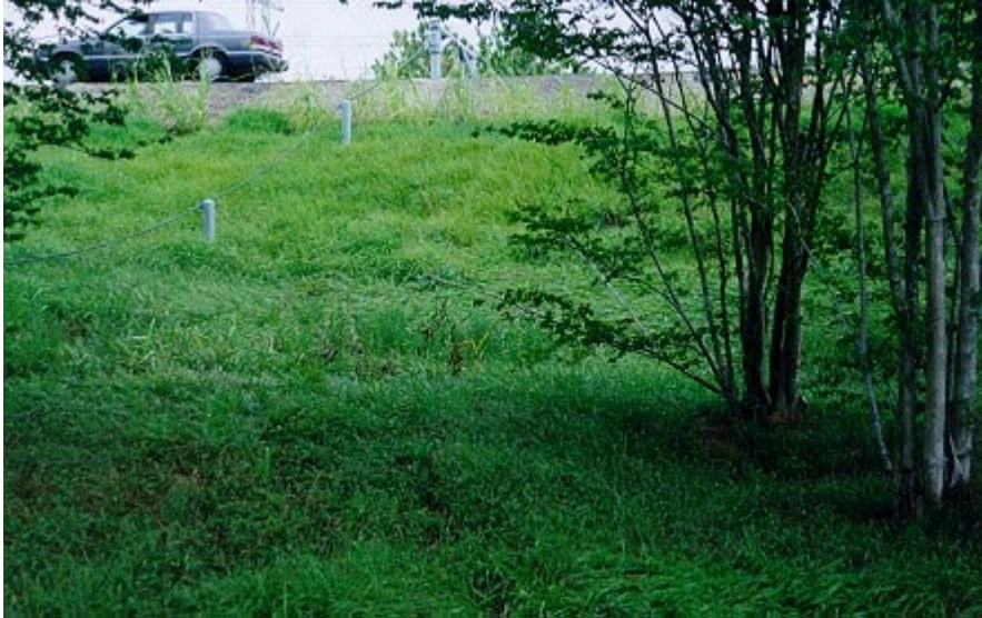
Figure 3.5: View of berm from inside Addicks Reservoir
