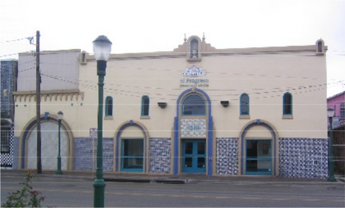
Figure 3.8: El Progreso Community Center, Guadalupe St., San Antonio, TX (Photograph by author).
