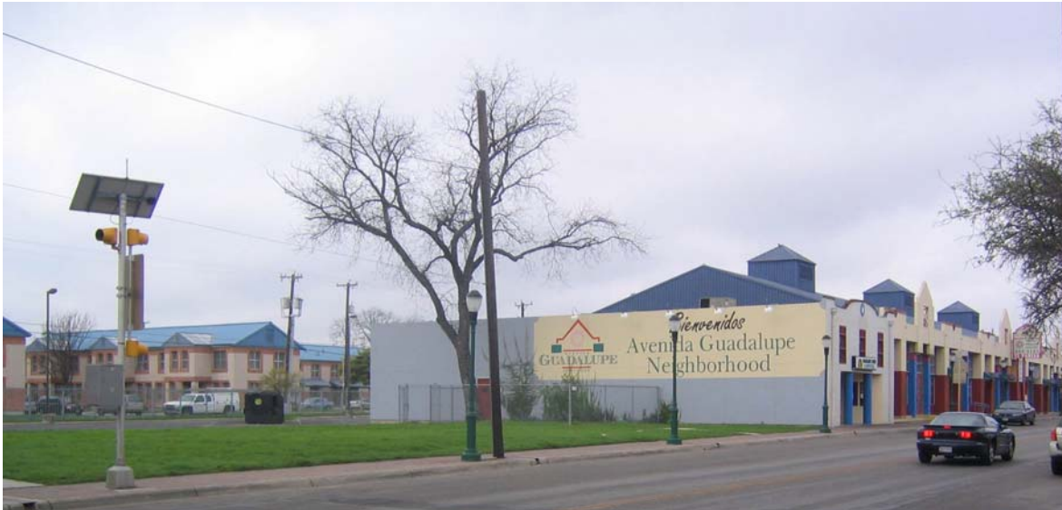
Figure 3.6: Entrance to Guadalupe Neighborhood, Alazan-Apache Courts visible on the left (photograph by author).
