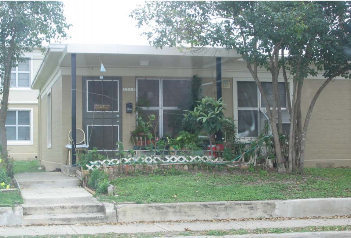
Figure 3.9: Single-story house with garden, Lincoln Heights, San Antonio, TX (photograph by author).
