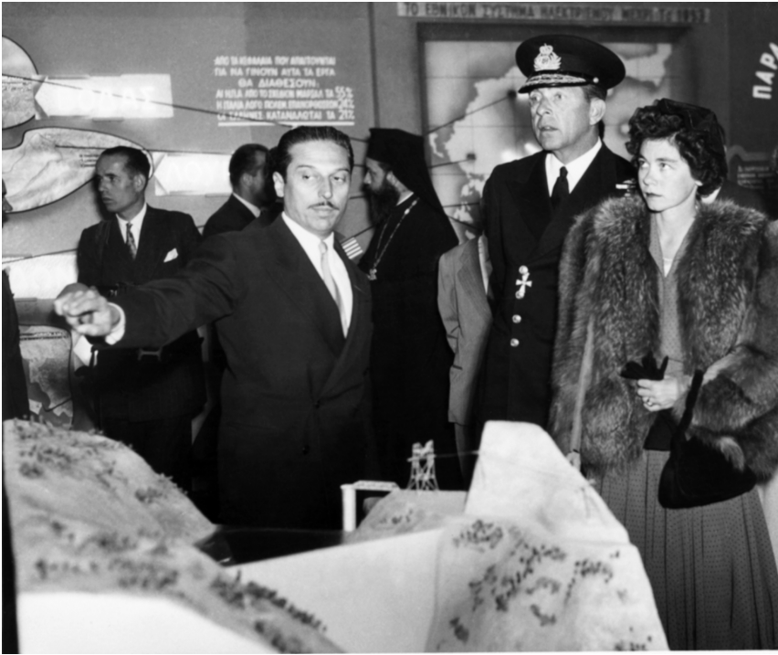
Fig. 4. Constantinos Doxiadis (left) in conversation with King Paul and Queen Frederica at the Athens opening of the “Electricity and Recovery” exhibition, 3 May 1950. Doxiadis Archives, Athens © Constantinos and Emma Doxiadis Foundation
