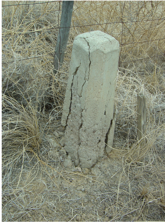
Figure 5-11: ROW marker deteriorating in west Texas.
