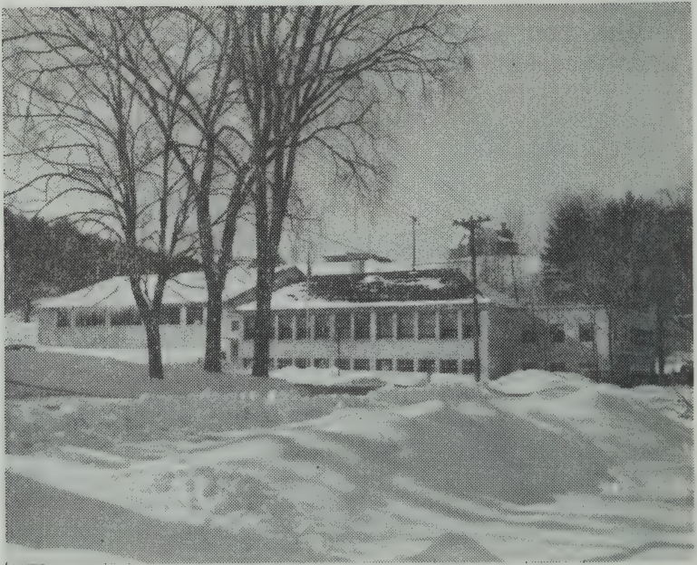
Front view of the new School
