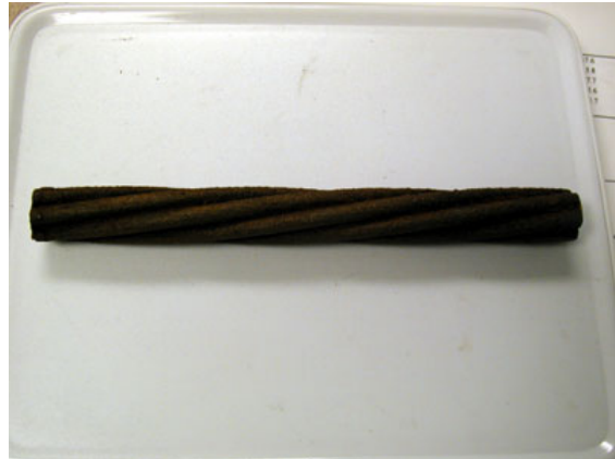
(b) After cleaning with wire brush
