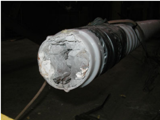
(c) Collapsed section (toward duct)
