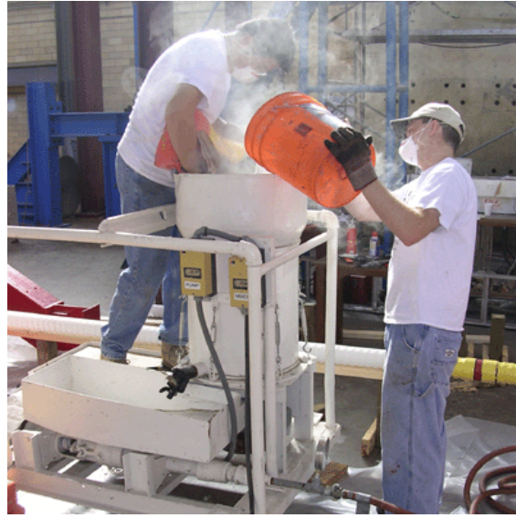
(b) Grout mixing and pumping
