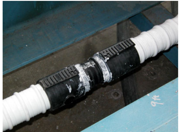
(b) Assembly of duct
