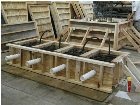
(c) Concrete form
