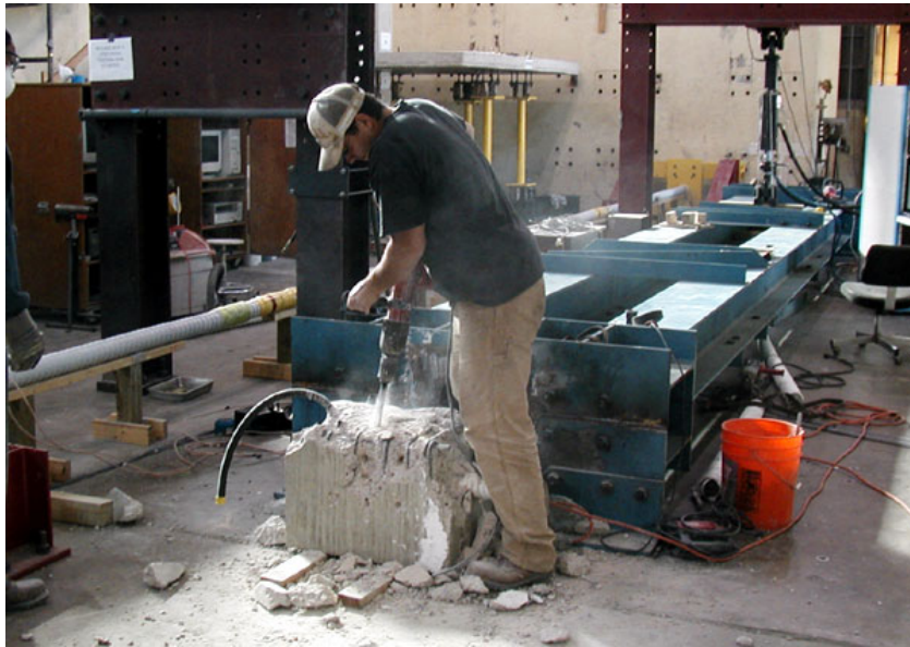
Figure 5.23 Demolition of Concrete Anchor Block for Tendon 01
