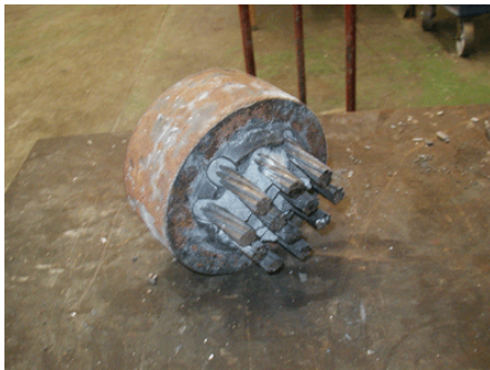
(c) Strands and wedges (south)
