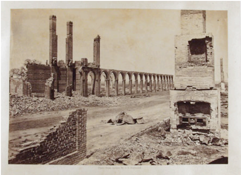
Figure 5: Barnard's "Ruins of the Railroad Depot, Charleston, S.C."
