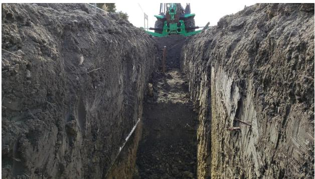
Photograph 25 – Parallel steel and PVC rural water supply lines within BHT 1, view to the south.
