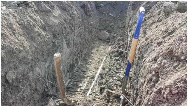
Photograph 22 – Two-inch steel rural water supply line encountered at 110 cmbs in BHT 1, view to the south.
