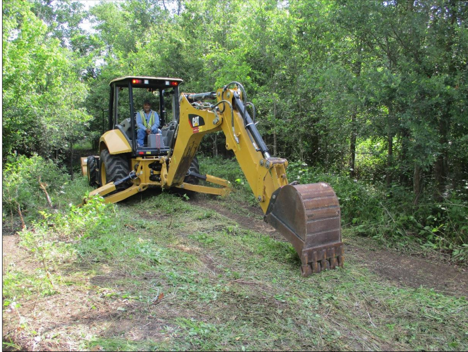
Figure 5. Backhoe and operator beginning excavation of trench BT1.
