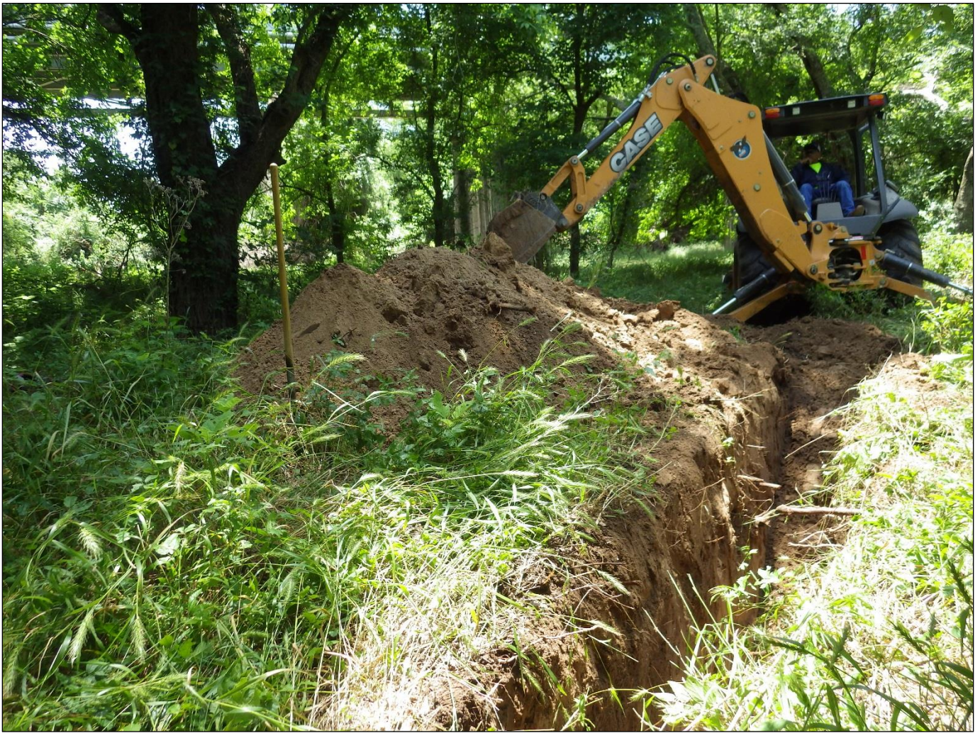
Figure 24. Excavation of BHT 3 in southwest quadrant of APE.
