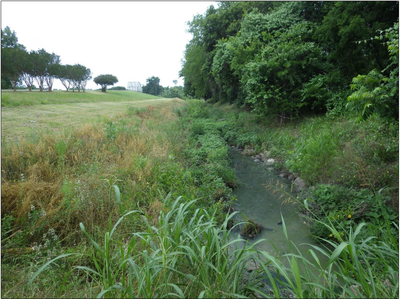
Figure 12. Stone-lined drainage ditch within APE, northeast quadrant.
