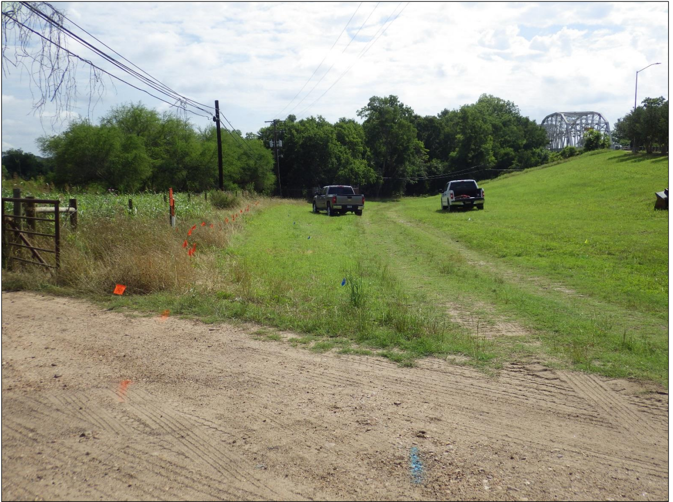
Figure 11. Steep bridge approach (right frame) on west side of river with buried utilities within APE, southwest quadrant.
