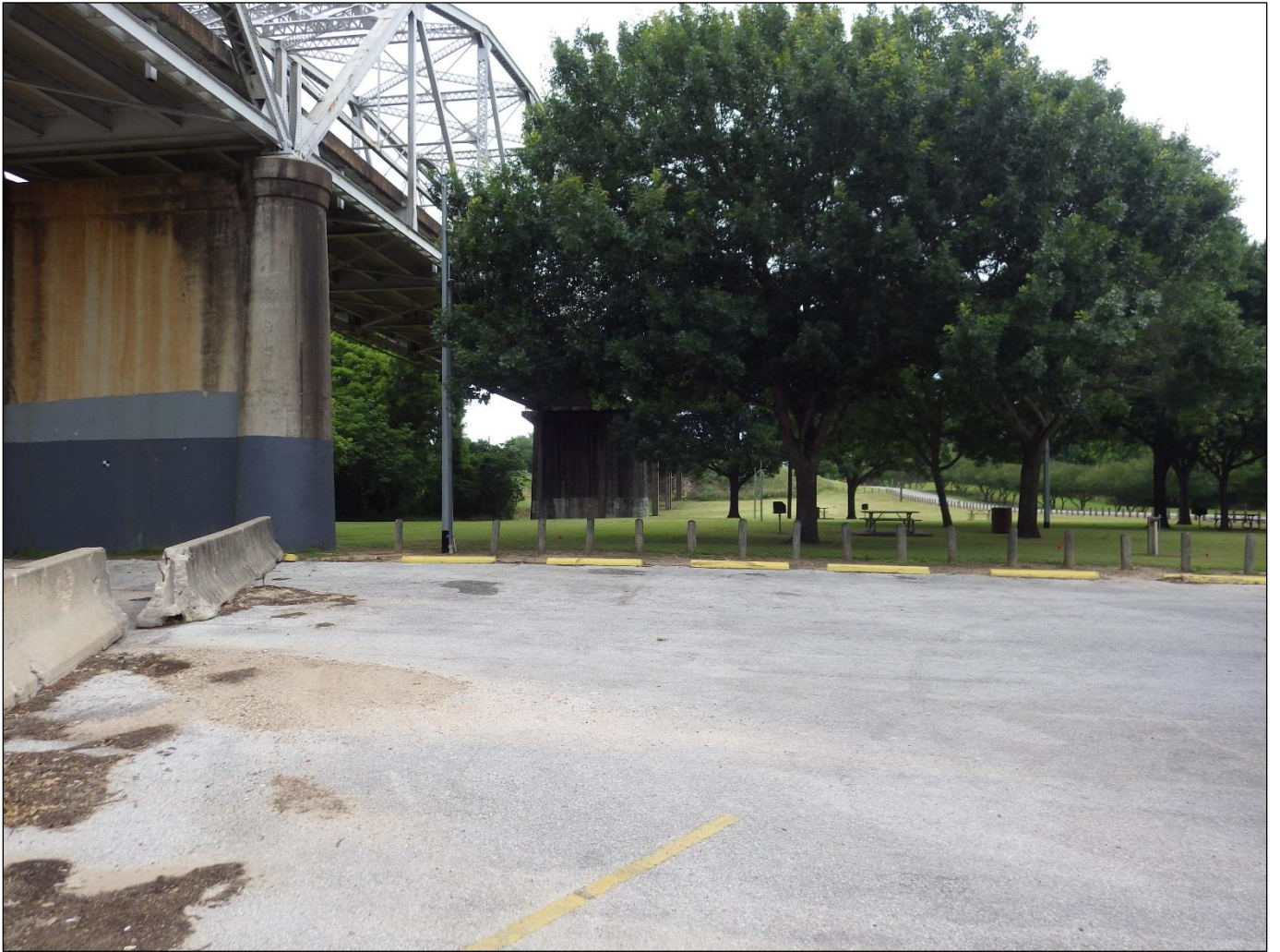
Figure 15. City park and parking lot beneath BS71E bridge within APE, southeast quadrant.
