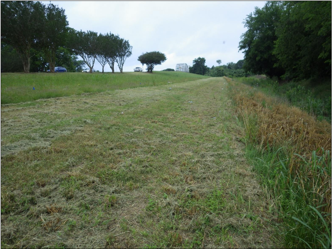
Figure 13. Steep bridge approach on east side of river, northeast quadrant.
