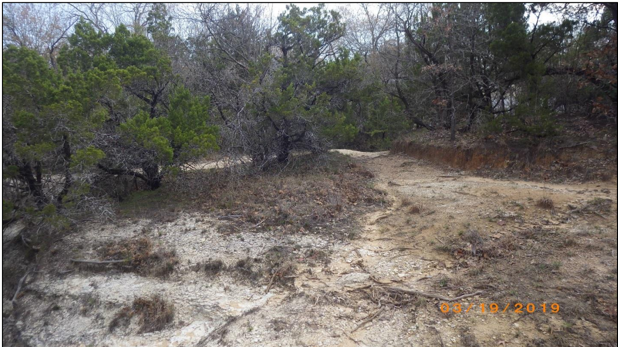
Figure 6. Erosion of shallow subsoils to bedrock along the east bank of Prairie Creek. View is to the north.
