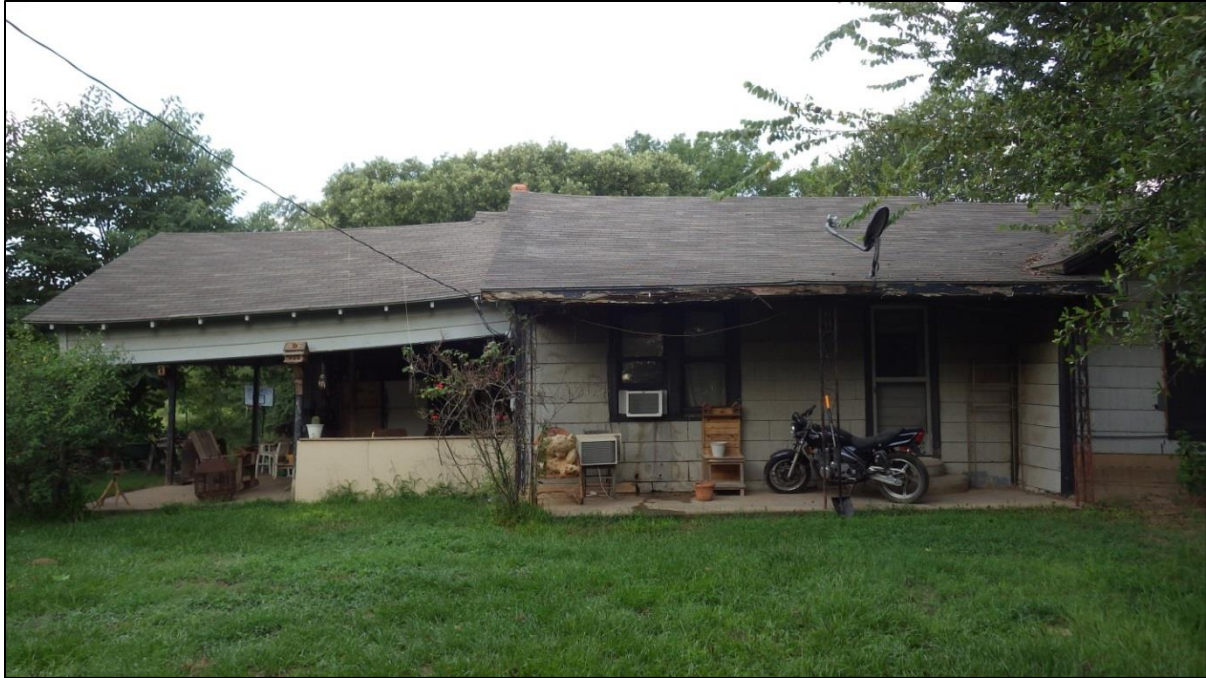
Figure 30. West-facing view of the house at site 41FN254.
