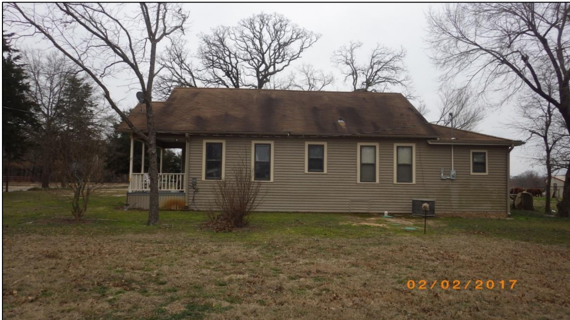
Figure 39. South-facing view of the house at site 41FN257, showing the hipped-roof addition on the house's west side.
