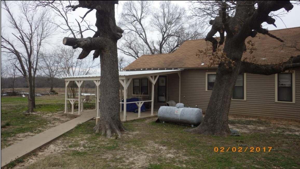
Figure 40. View looking northwest at the site 41FN257 house, showing the covered porch and gable-roofed addition on the house's west face.
