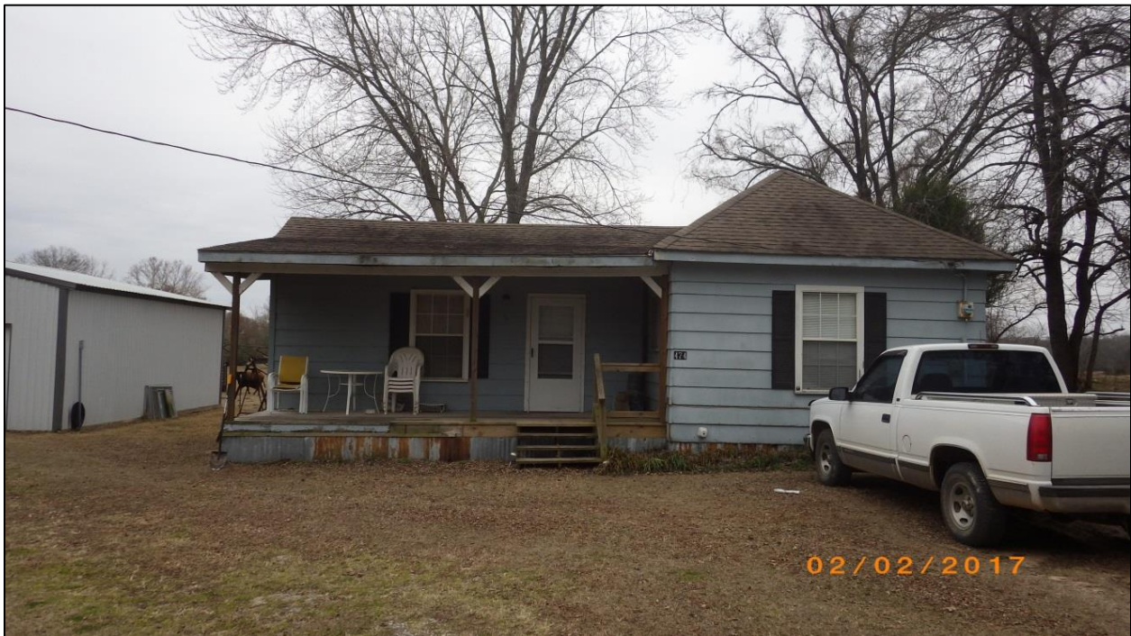
Figure 33. South-facing view of the house at site 41FN255.
