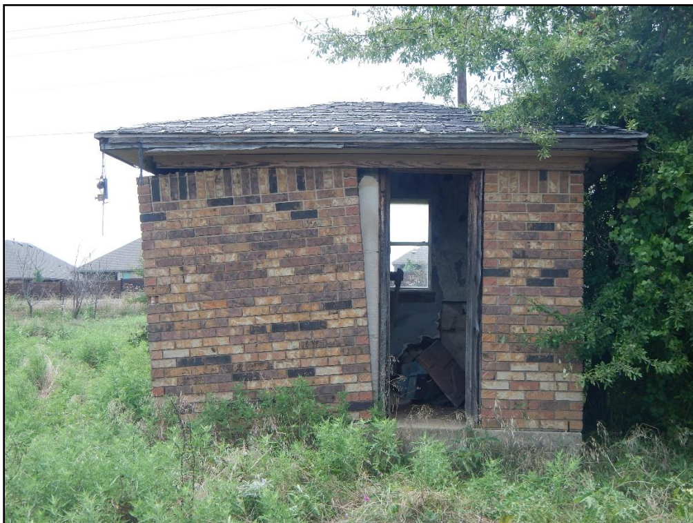
Figure 20. View of brick outbuilding showing the entrance and window; view west.
