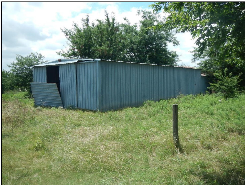
Figure 26. View of the northern end of the barn; view southeast.
