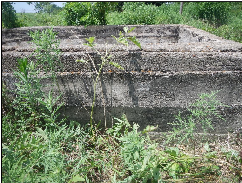
Figure 22. South wall of the concrete box showing construction method; view north.
