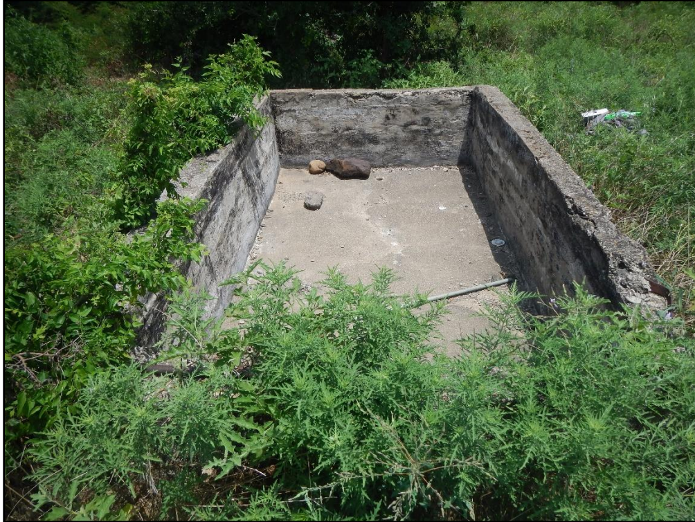
Figure 21. View of concrete box showing the depth; view east.
