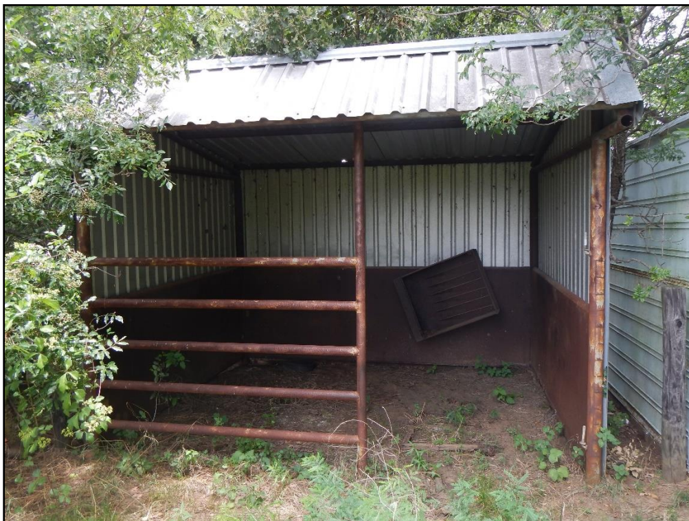
Figure 24. View of shed 2 showing the open western side; view east.
