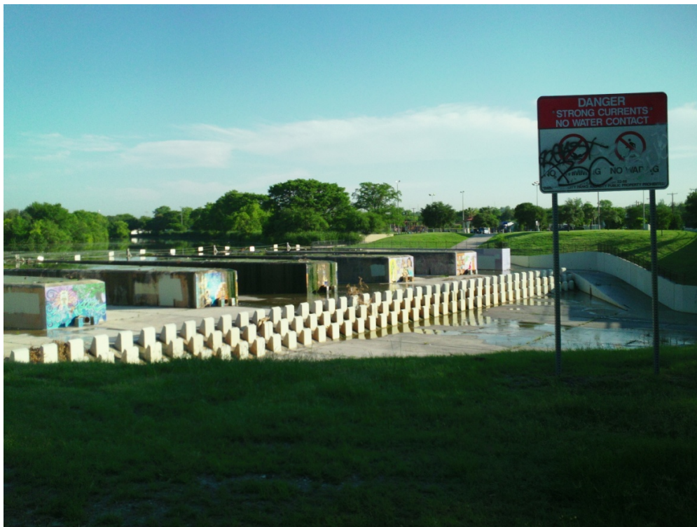
Figure 12: Overview of dam, facing north from southeast project terminus.
