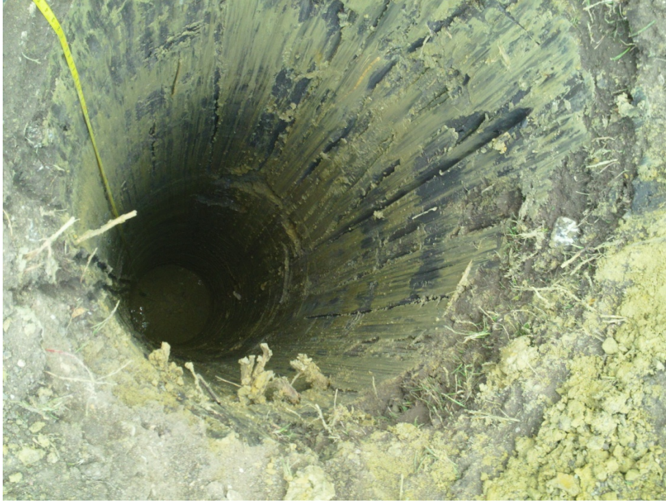
Figure 23: Pier drilling at completed depth.
