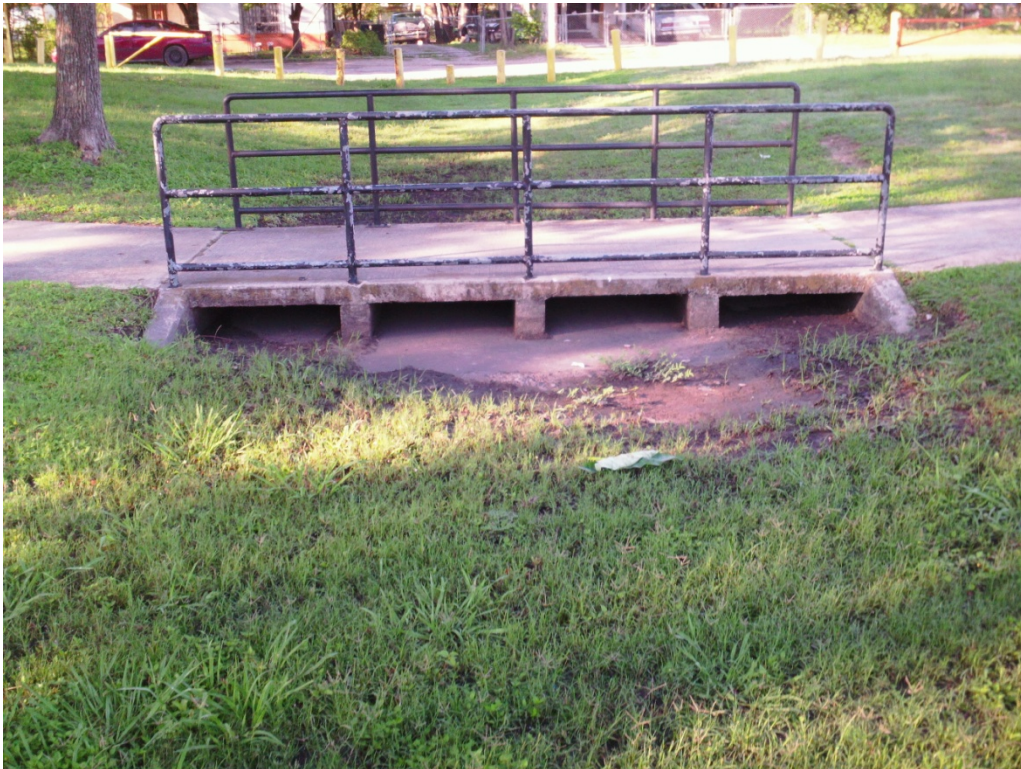
Figure 14: Overview of footbridge and culvert ditch drainage, facing south.
