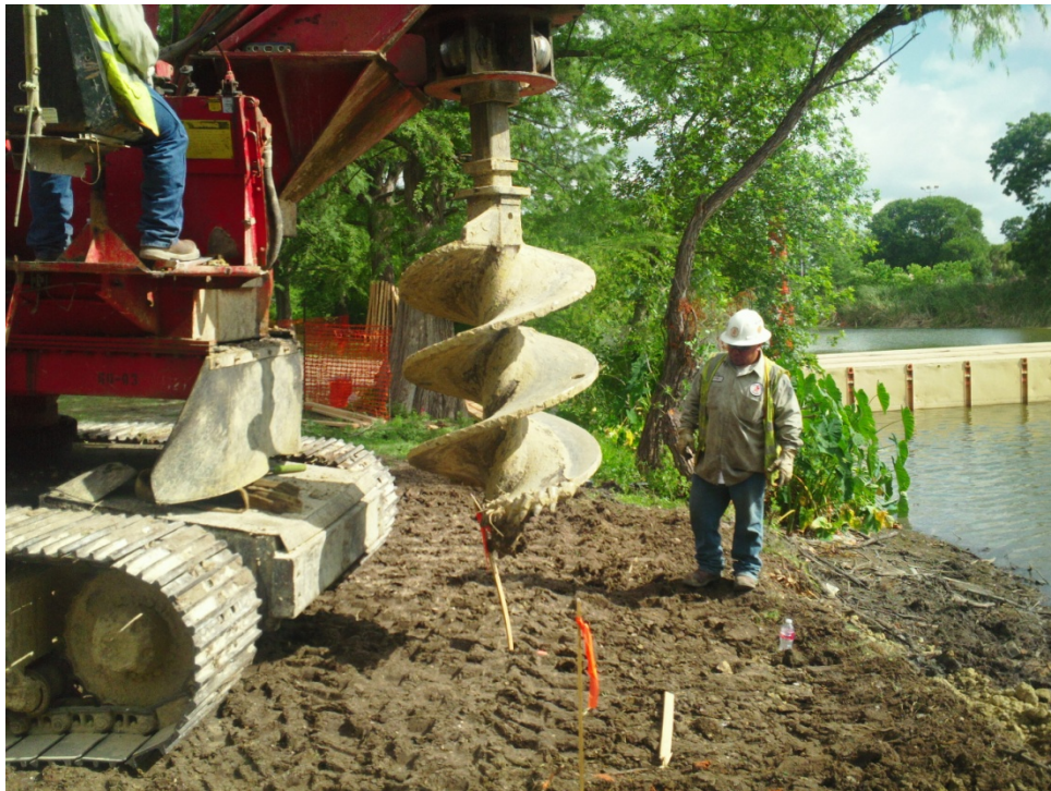
Figure 24: Pier drilling underway.
