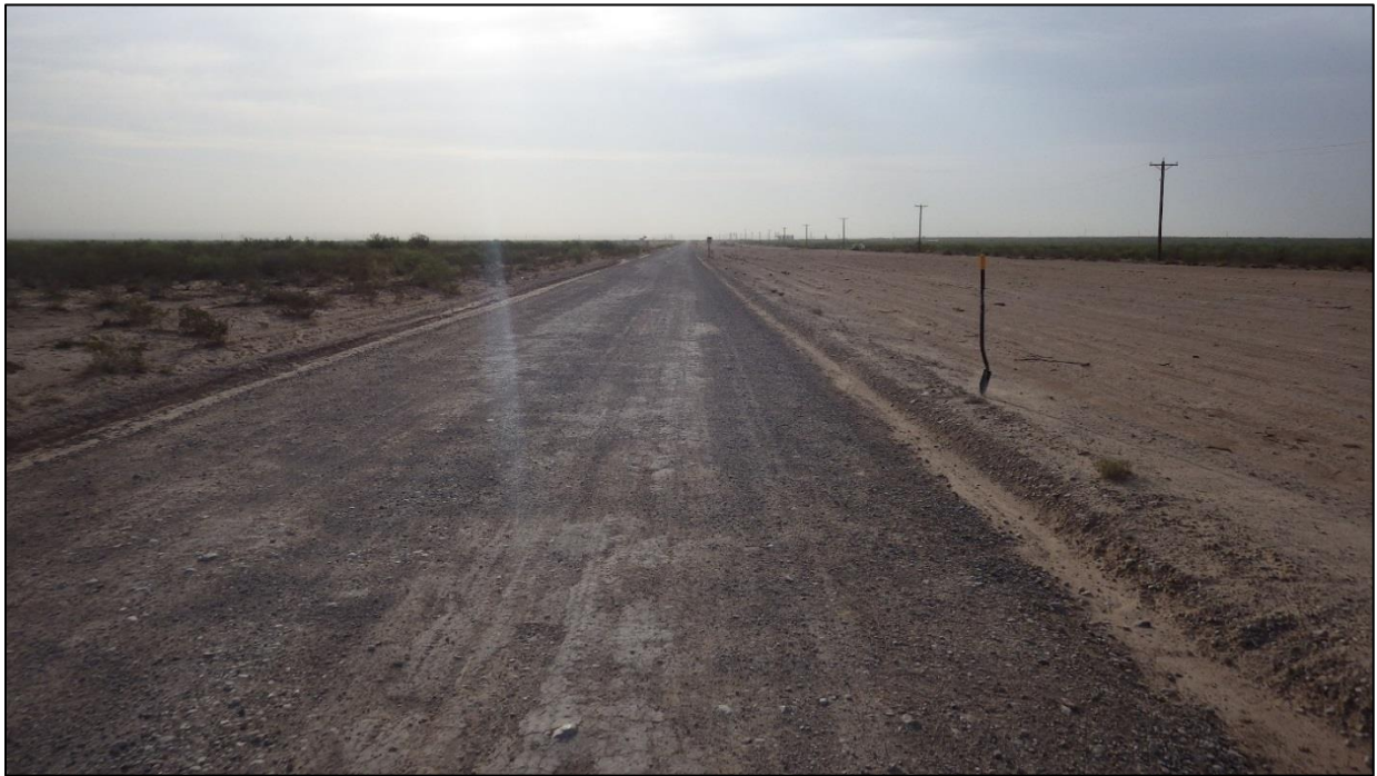
Figure 9. Gravel road and pipeline installation that cross into the ROW, photo taken facing east.
