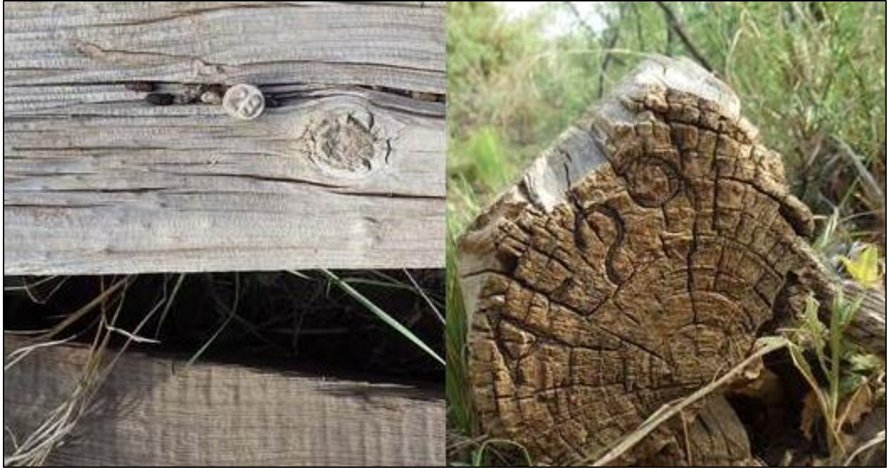
Figure 22. Diagnostic features observed on discarded railroad ties. Left: date nail with number "28" on a round head. Right: "AE29" brand on end of railroad tie.
