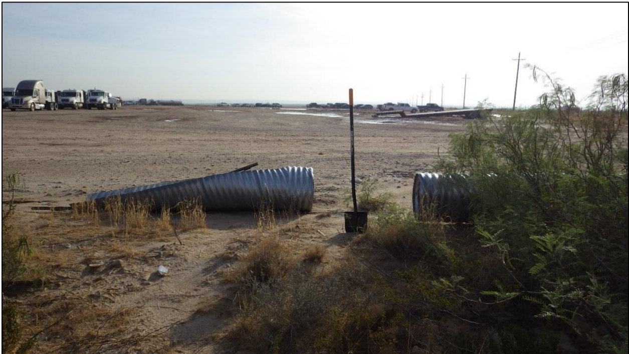
Figure 17. View of where the route crosses into the parking lot on the north side of SH652, photo taken facing northeast.
