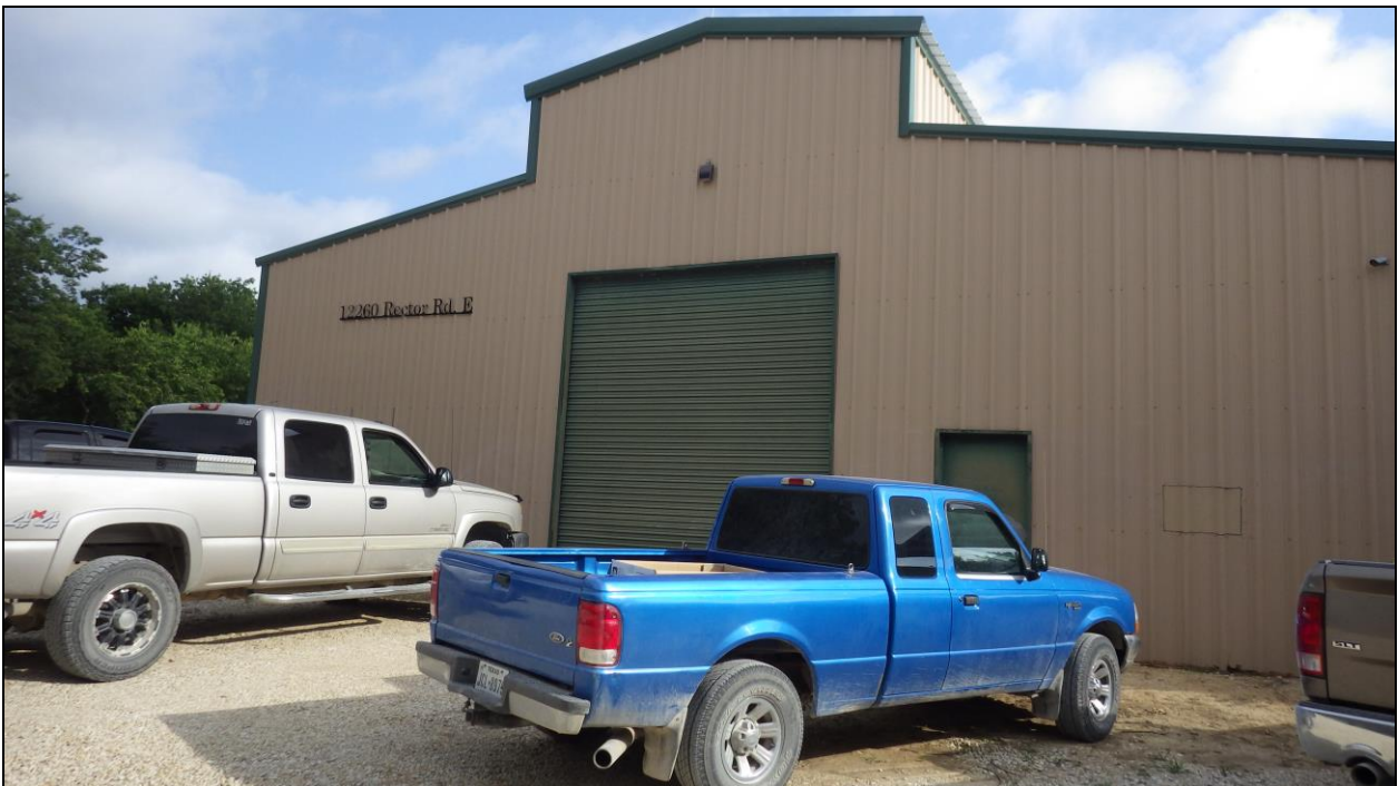
Figure 7. Barn located within the alternative route survey area. View is to the north.
