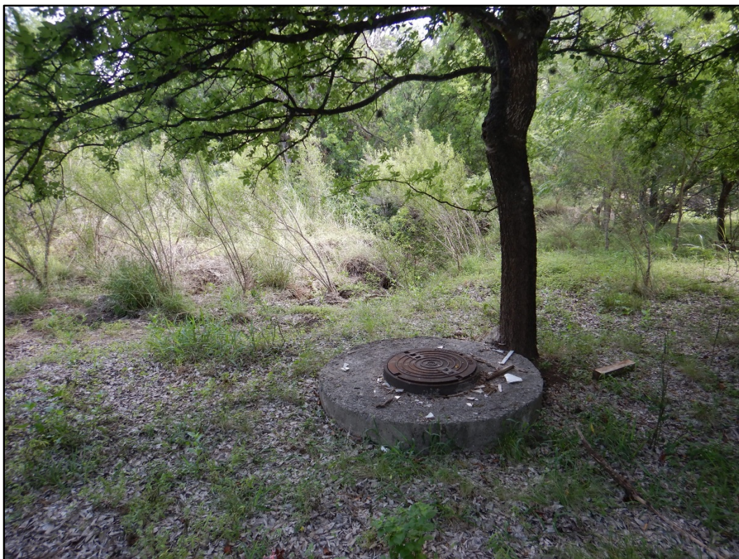
Figure 11. Photograph of sewer line cap along the drainage at north end of project area, facing northeast.
