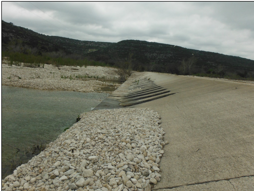
Figure 8. Bridge-class culvert at the Nueces River crossing, facing north.
