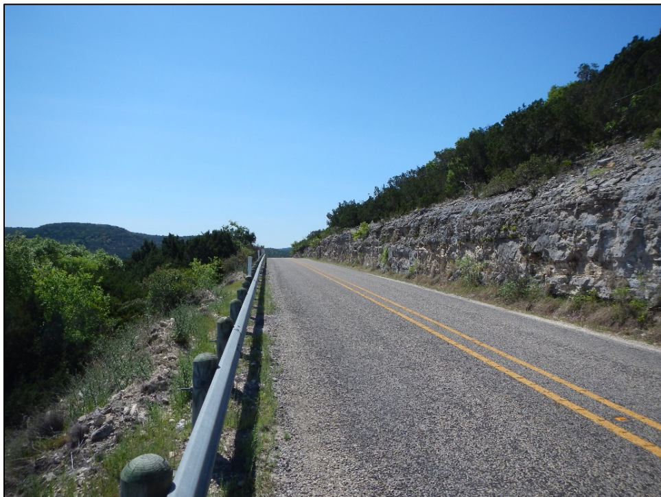
Figure 6. Typical road cut through limestone bedrock, facing south.
