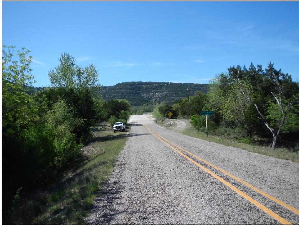
Figure 7. Typical elevated roadway conditions with driveway disturbances, facing northwest.
