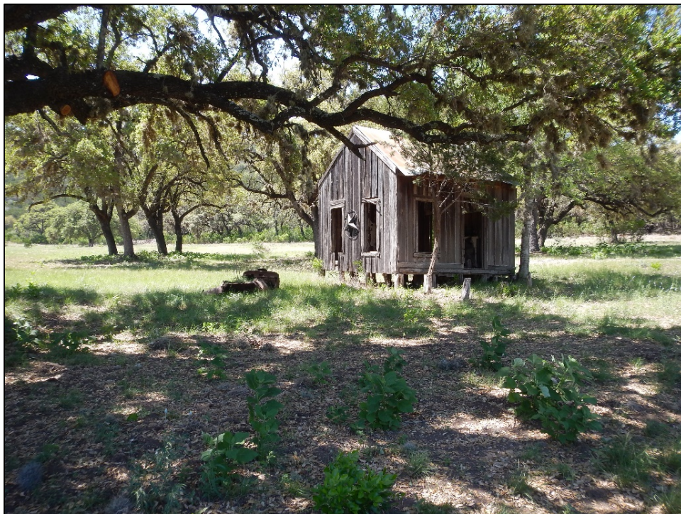
Figure 9. Overview of historic-age cabin immediately adjacent to the Survey Area, facing west.
