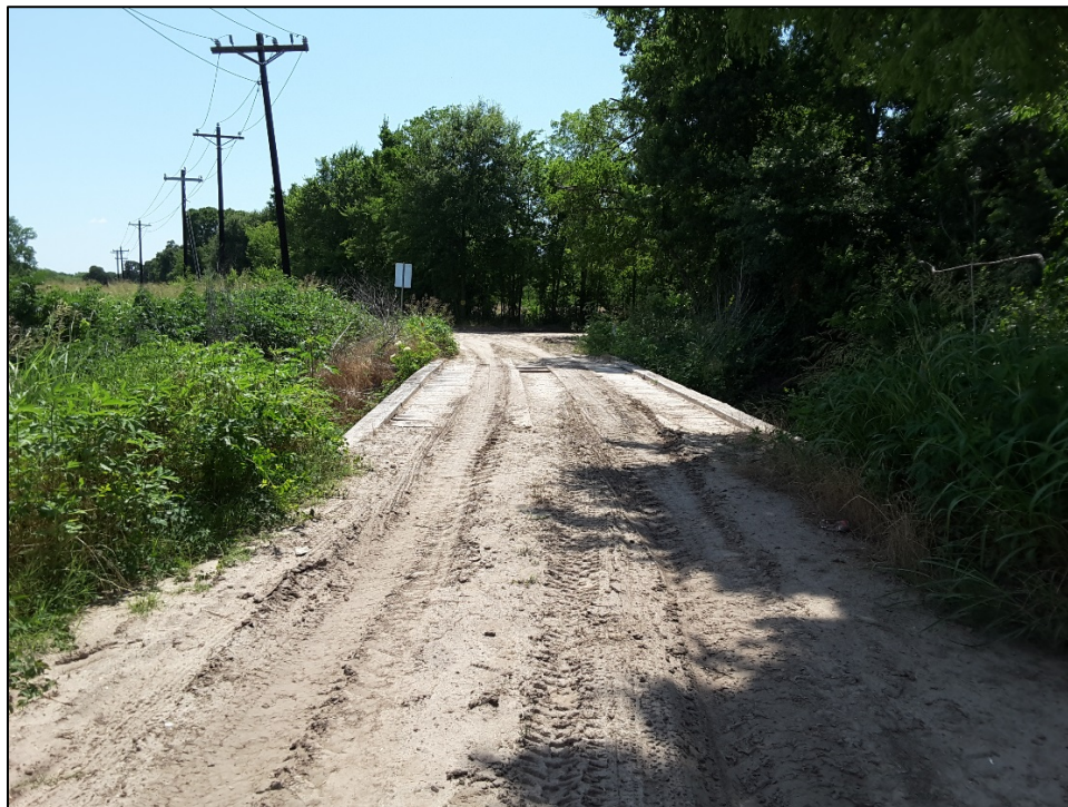
Figure 6. Overview of CR 279 showing bridge to be replaced, facing west
