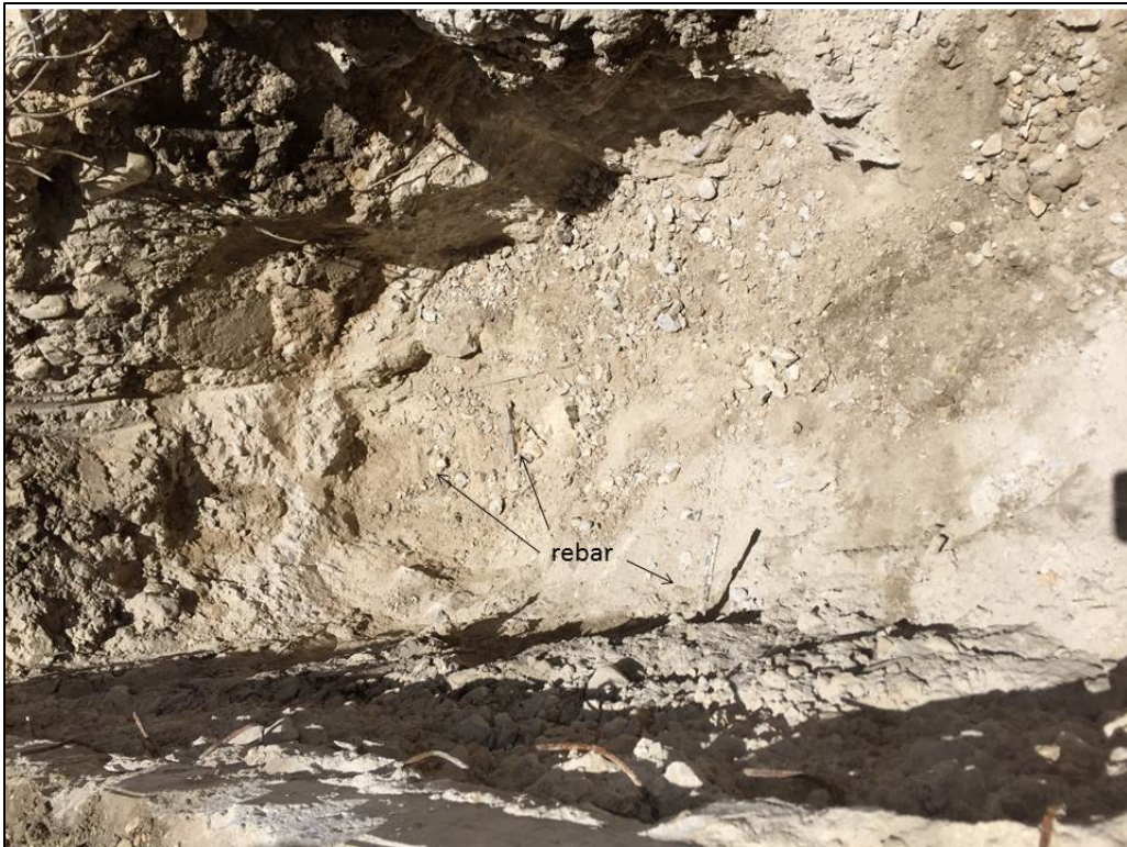
Figure 9 Rebar in trench closest to the building
