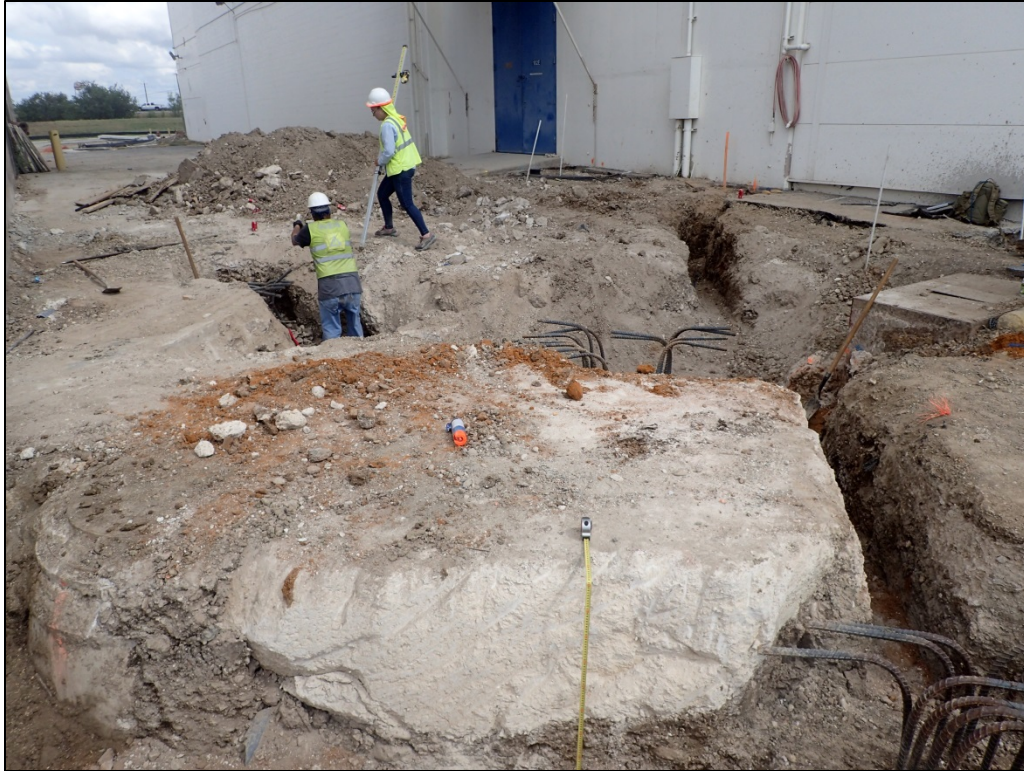
Figure 11 Overview of Wall 3 and utility trenches showing caliche layer facing north
