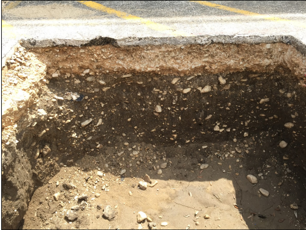
Figure 6: Typical trench profile for Wall 1 facing east
