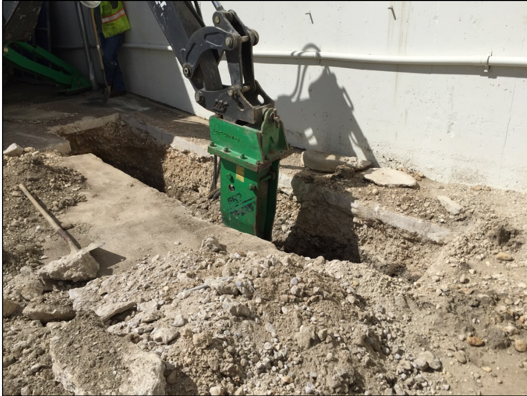
Figure 5 Backhoe digging trench for Wall 2
