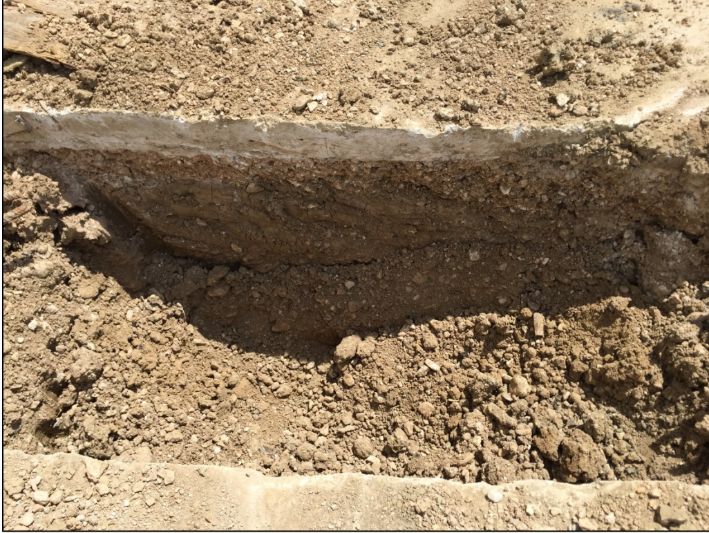
Figure 8 Trench 9 profile (Wall 2) facing east
