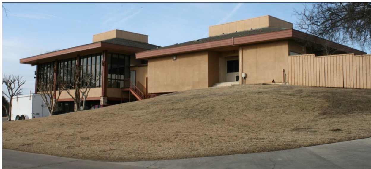
Figure 12. East elevation of center wing and east and north elevations of north wing. View looking southwest.
