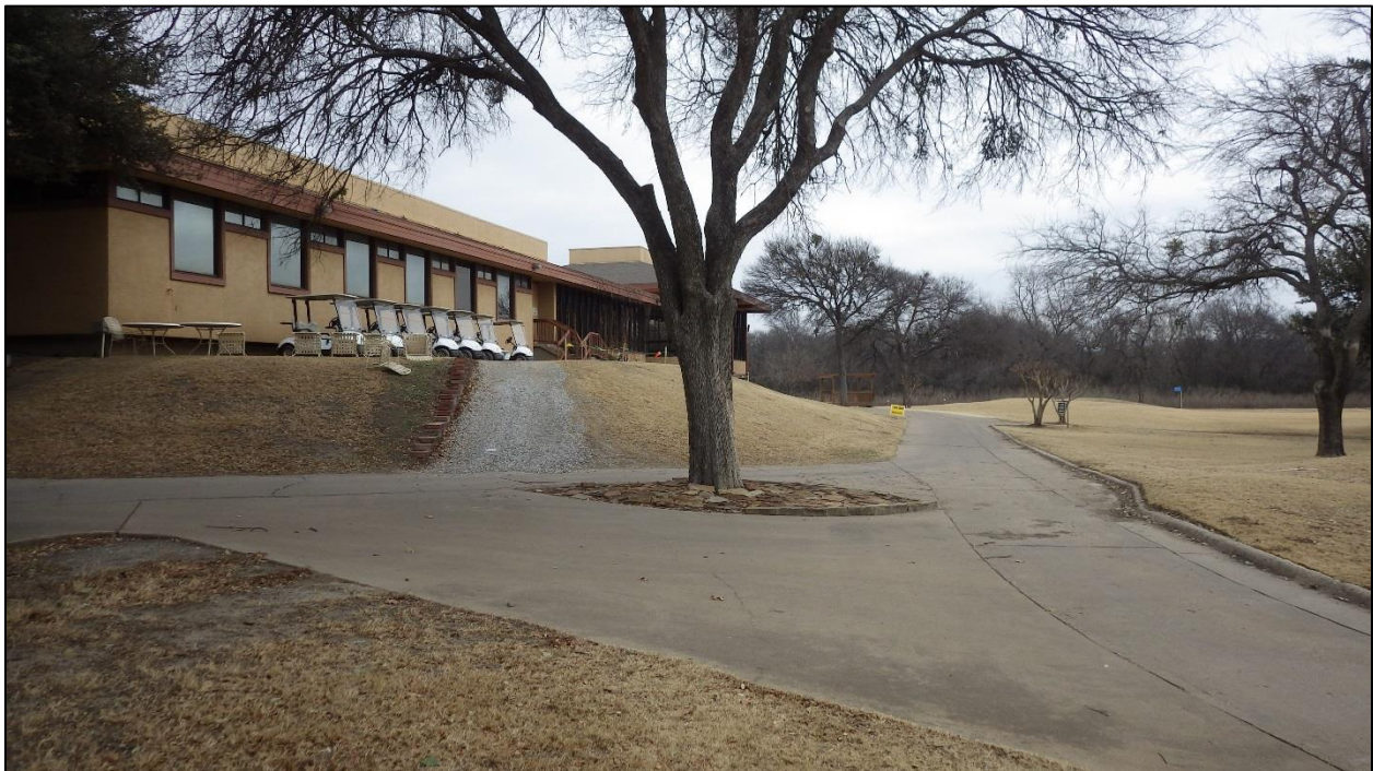
Figure 25. Area D is left of the path with golf carts part on top of it, view to the east.
