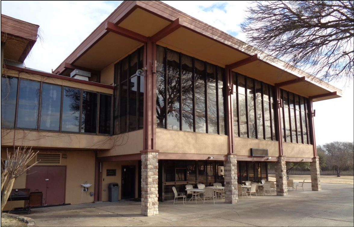
Figure 10. South elevations of link and center wing. Note how the lower level is recessed under the upper level. View looking northeast.
