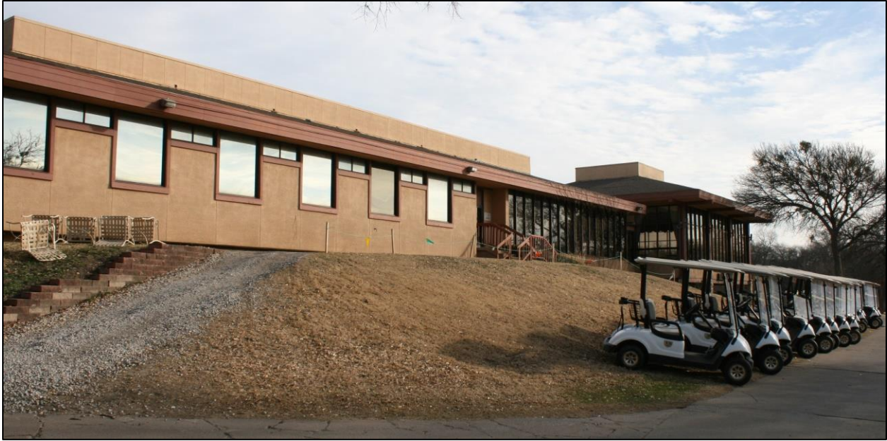
Figure 9. South elevation of west wing. Looking northeast.
