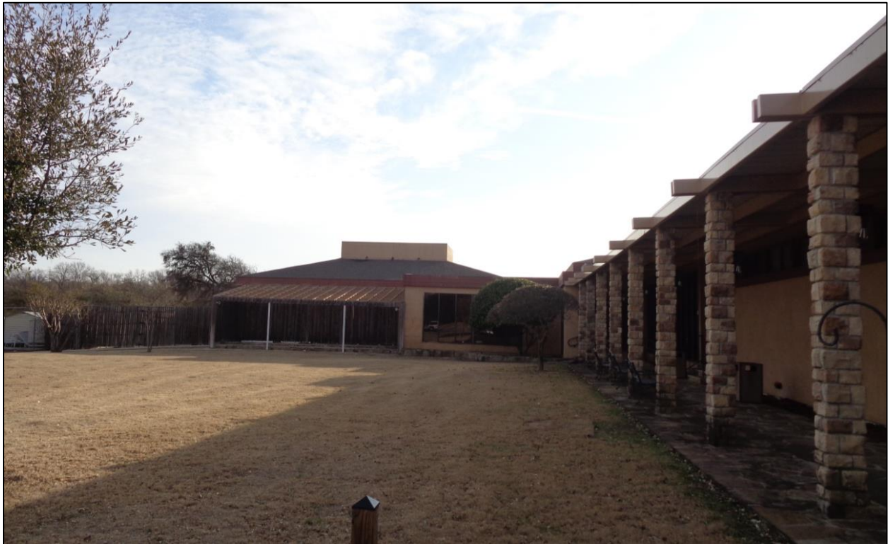
Figure 8. West elevation of the north wing and canopy along north elevation of west wing. View looking east.
