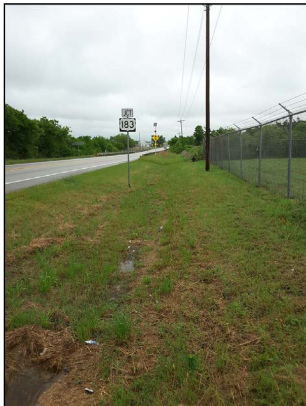
Figure 8. Overview of approach along FM 1625 to bridge spanning North Fork Dry Creek, facing northwest.
