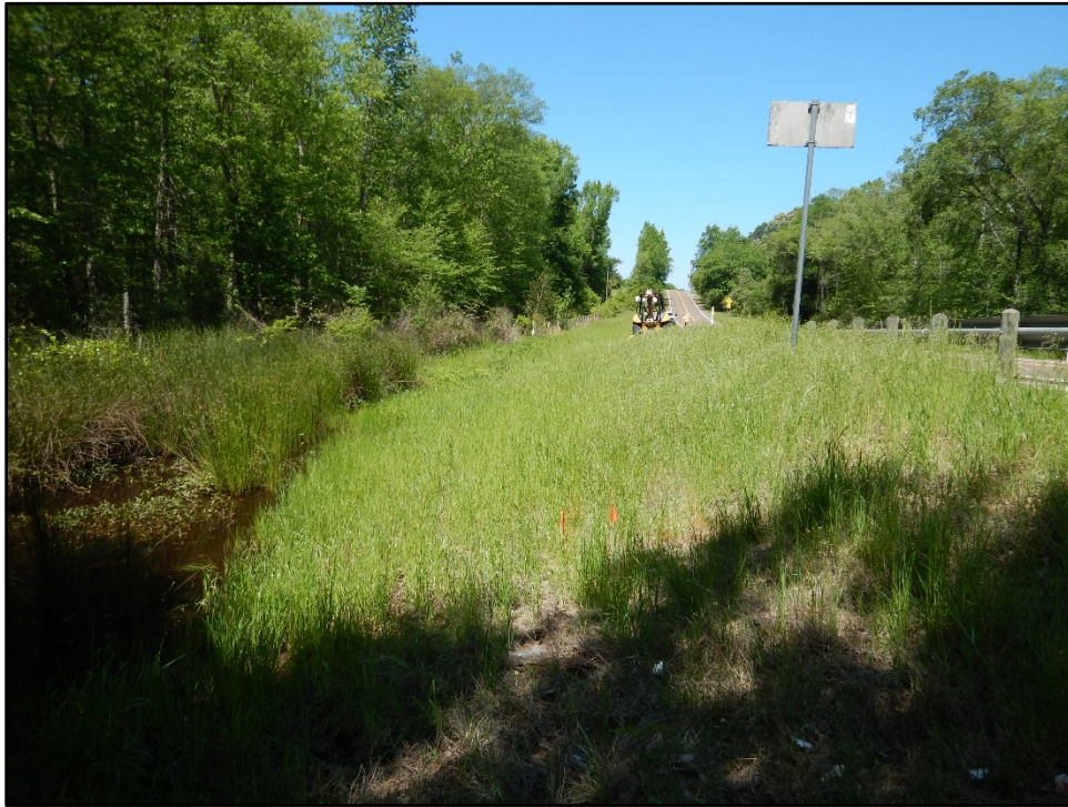
Figure 6. South side of FM 1511, on the west bank of Resaca Creek, with flagged utilities in foreground, standing water wetlands (left), and backhoe at BHT1 location, facing northwest.
