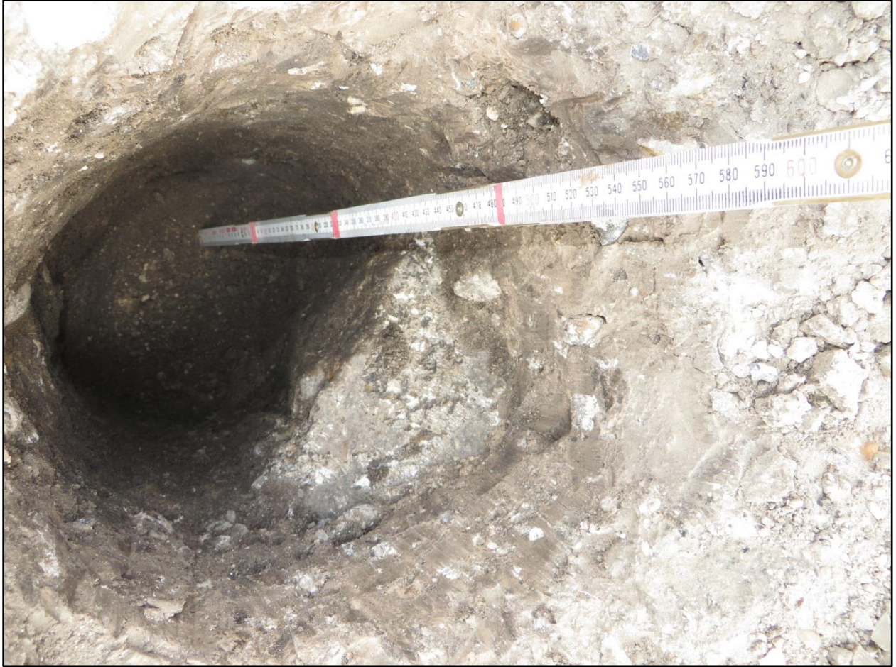
Figure 5-5. Large fragment of concrete in southwest wall of ST 4, approximately 20-cmbs.
