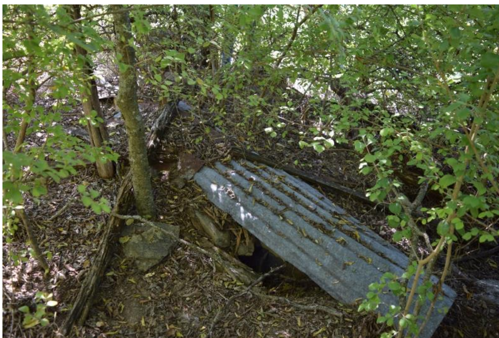
Photo 18. 41PR163/41PR164, possible well house over possible well.
