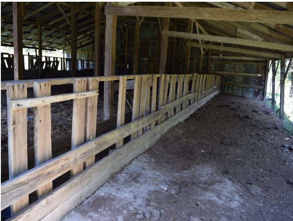
Photo 27. 41PR166, detail of milking area in milking barn.
