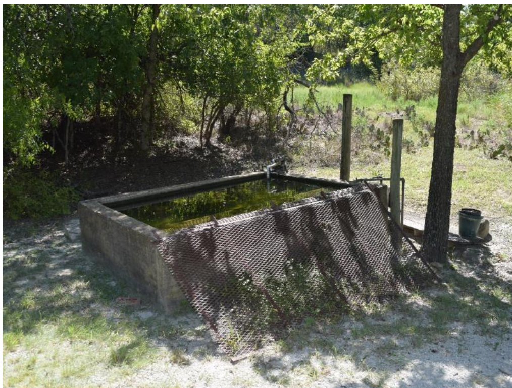
Photo 20. 41PR163/41PR164, concrete water trough.
