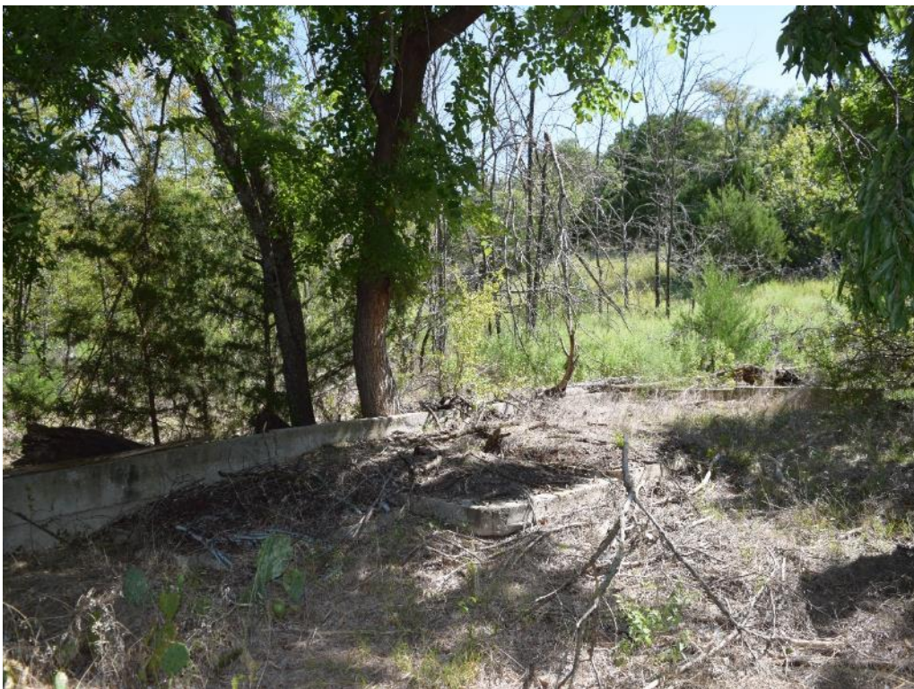
Photo 15. 41PR163/41PR164, milking barn foundation.
