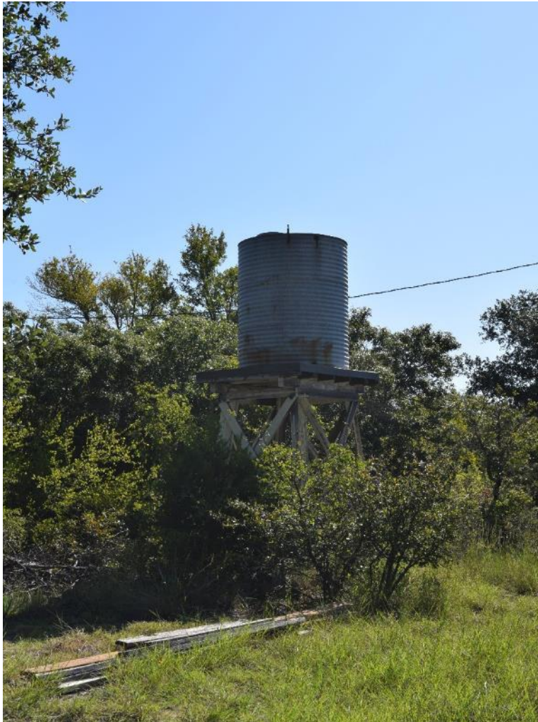
Photo 12. 41PR163/41PR164, water tank.
