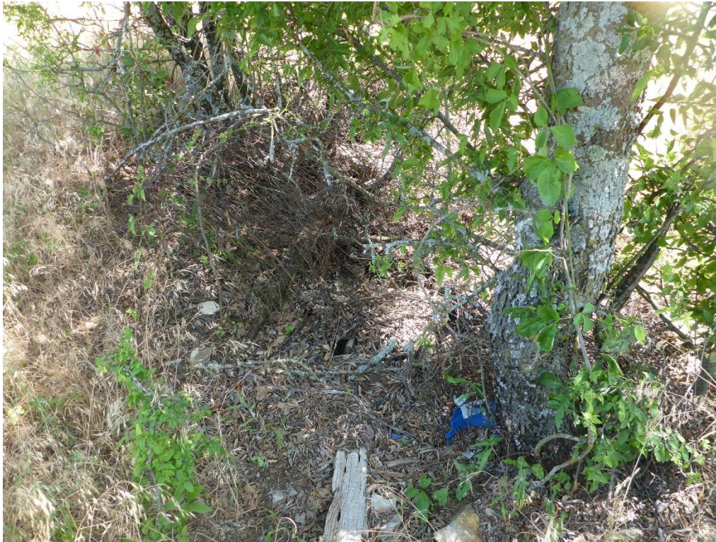
Photo 35. 41PR185, collapsed rock lined root cellar.
