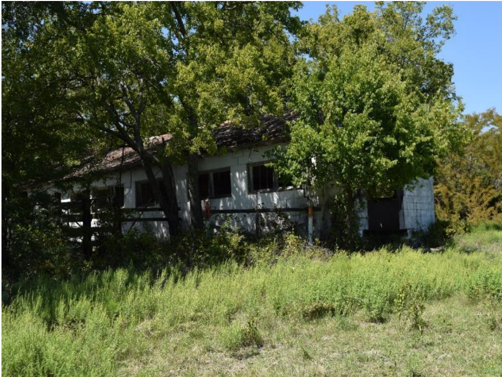
Photo 28. 41PR166, dairy barn and office.
