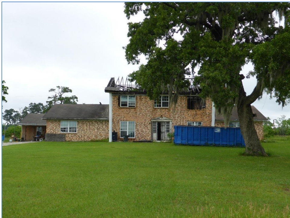
Figure 10. Abandoned, burned modern house north of Old Hempstead Road; view to the north.
