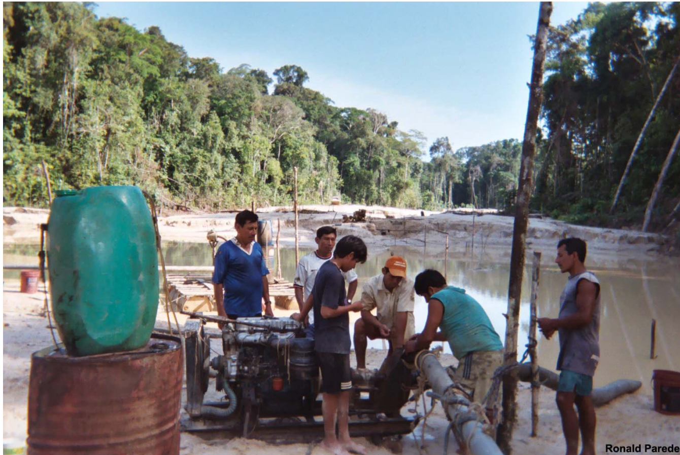
Figure 50. Hydraulic pumps are used to blast water at great pressure and destabilize the earth thus freeing the gold to settle on the bottom. The holding pool and mud/sand bars have replaced a small rainforest creek. Photo: Ronald Paredes del Águila.
