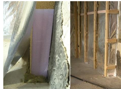
figure 45: Internal vapour barrier ©Eurac
