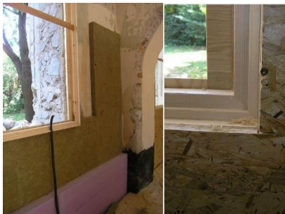
figure 46: Internal insulation (mineral wool) and OSB ©Eurac
