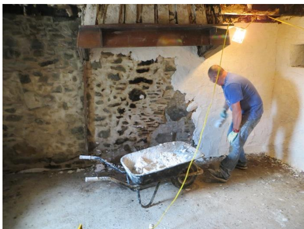
figure 21: First plaster coat being applied to the wall © HES
