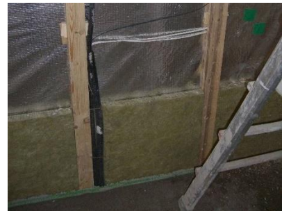
figure 48: Installation layer ©Eurac
