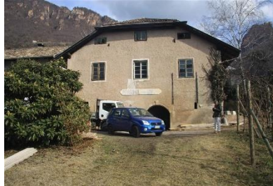
figure 24: Front of the building pre- renovation © Eurac
