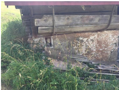
Old wall before renovation © Gehret Design
