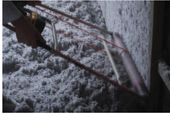
figure 19: Flattening the cellulose material prior to attaching the plasterboard © HES
