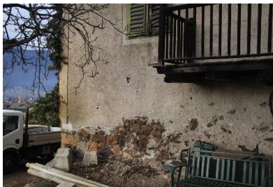
figure 26: Detail of the building pre renovation © Eurac
