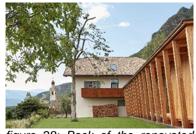
figure 28: Back of the renovated building © René Riller
