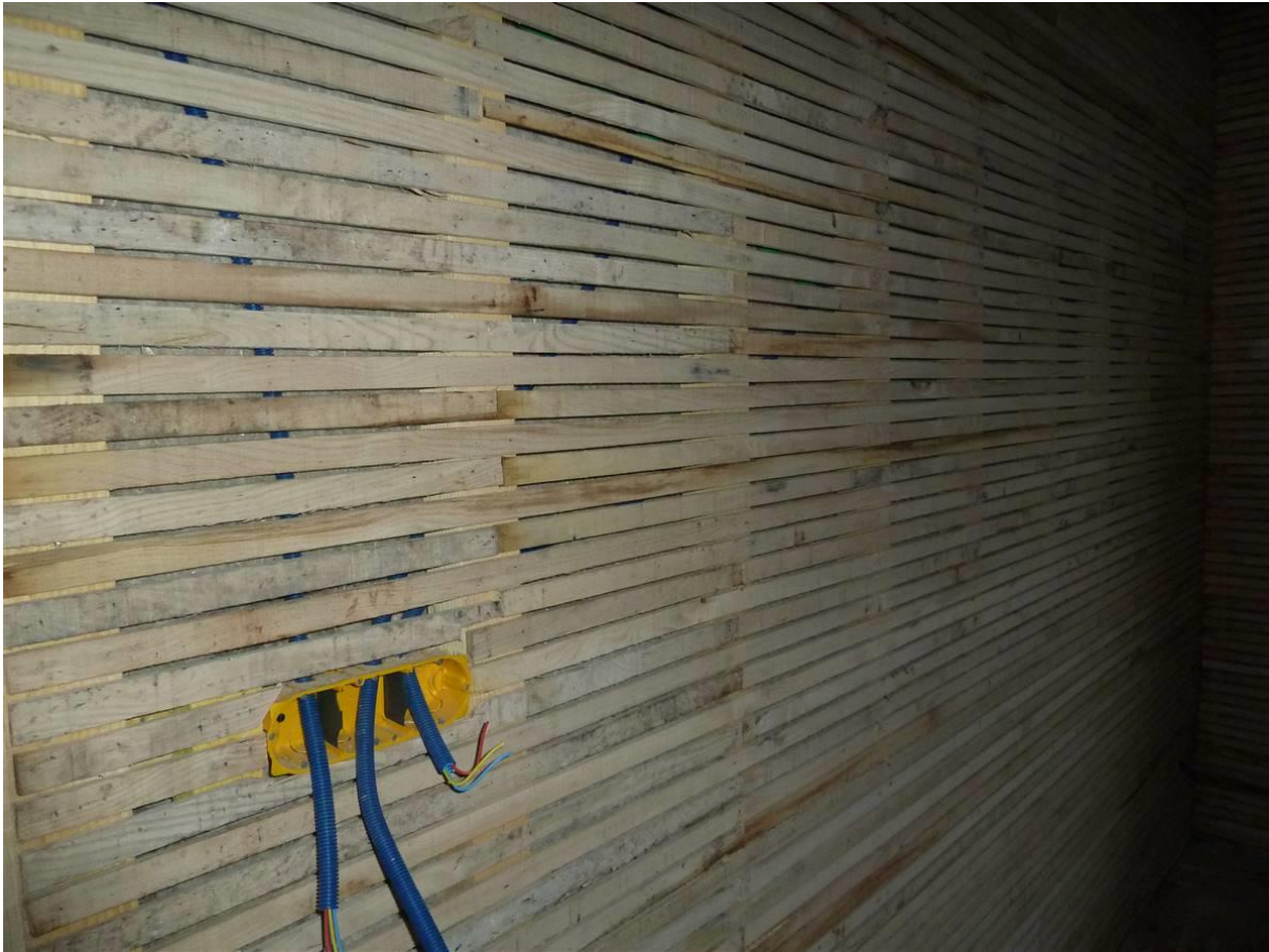
figure 164: Chestnut laths as a support for the earth render
