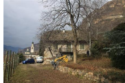
figure 25: Side of the building pre renovation © Eurac
