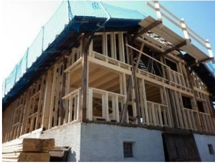
figure 167: Construction phase, © Familie Schmölz
