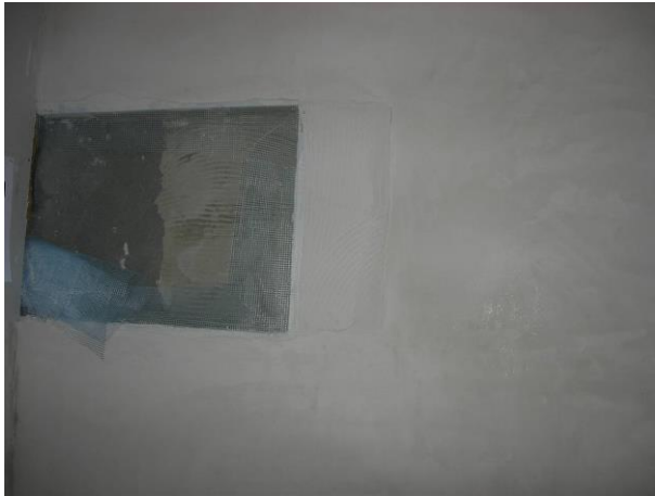
figure 41: The almost completely insulated wall using calcium silicate board © HES
