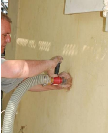
figure 78: Intervention to improve thermal insulation of external walls. © M. Hutterli
