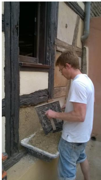
figure 161: Application of the hemp concrete from outside © Philippe Glé
