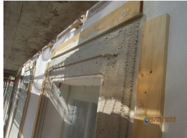
figure 127: Impressions from the work on the aerosol insulated façade, © Trimmel Wall Architekten ZTGmbH
