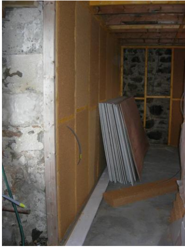
figure 38: A finished wall with the wood fibre board insulation © HES
