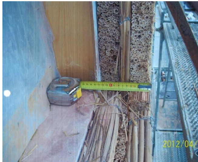
figure 138: Construction phase - external insulation thickness, © Hansjörg Plattner
