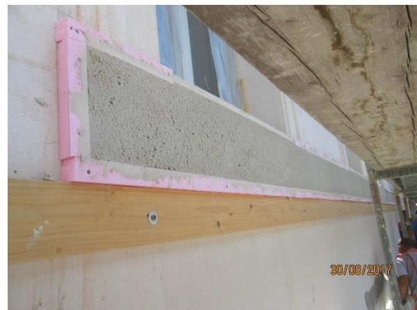
figure 131: Impressions from the work on the aerosol insulated façade, © Trimmel Wall Architekten ZTGmbH
