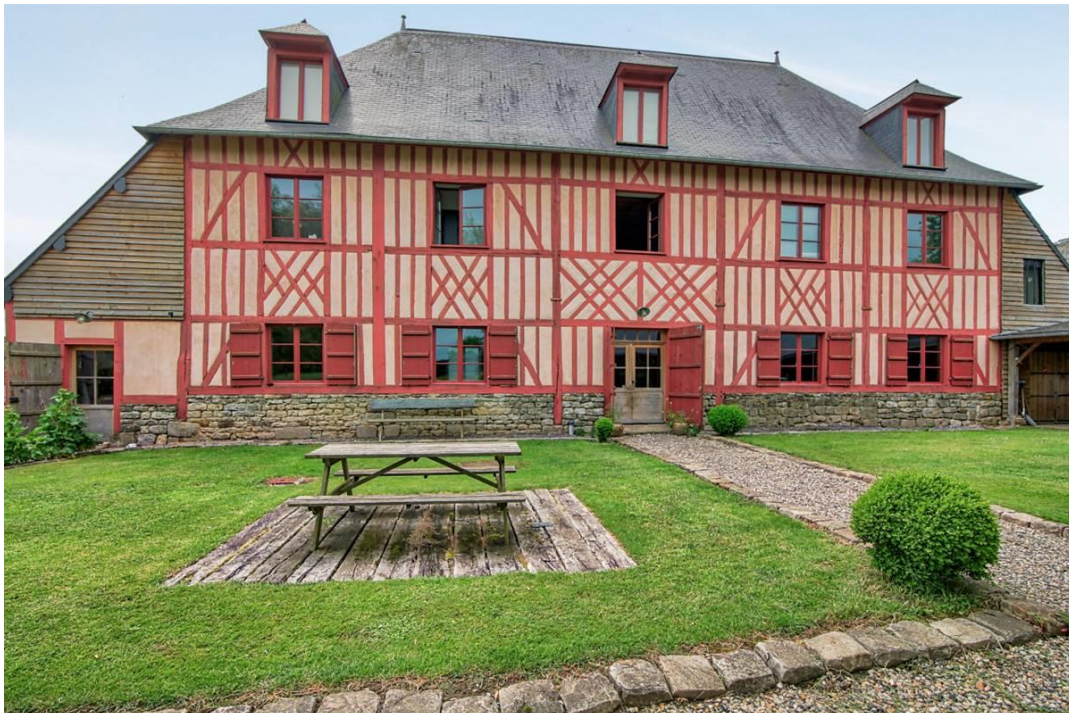
Figure 4: The internal insulated timber-framed barn (Cerema)
