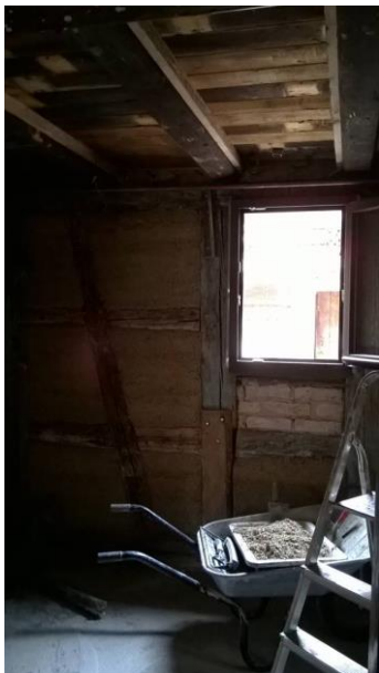
figure 160: Hemp concrete in place from inside, © Philippe Glé
