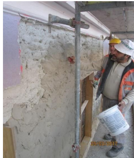
figure 125: Application of the aerogel plaster, © Trimmel Wall Architekten ZTGmbH
