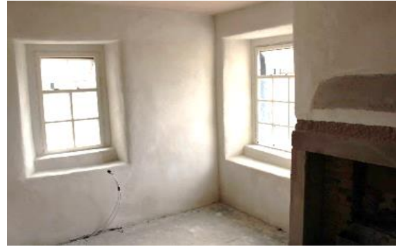
Figure 31 Insulated wall (lime plaster and cork) © Ecological Building Systems
