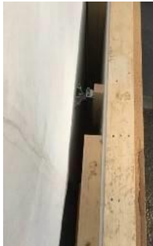
figure 154: Detail of the facade, © Michael Flach
