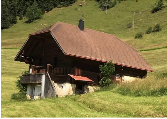
figure 146: Before renovation © Gehret Design
