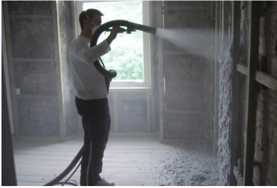
figure 18: Blowing on the wet cellulose insulation material © HES
