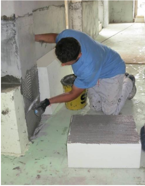
figure 6: Installation of internal insulation, © Eurac
