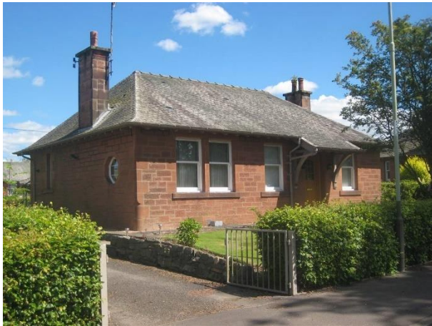
figure 88: View of the case study property © HES
