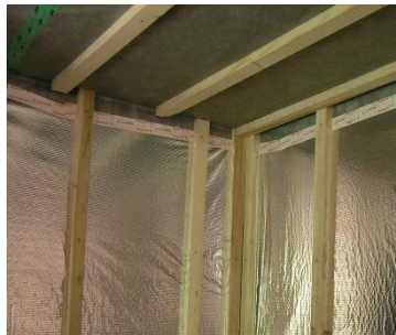
figure 47: Vapour Barrier and ceiling ©Eurac
