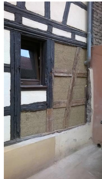
figure 162: Before application of the lime plaster © Philippe Glé
