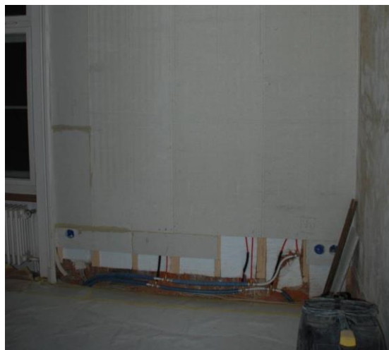
figure 75: Internal wall intervention © M. Hutterli
