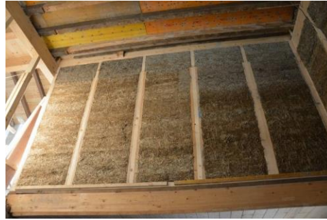
figure 168: Straw in stand construction, © Familie Schmölz
