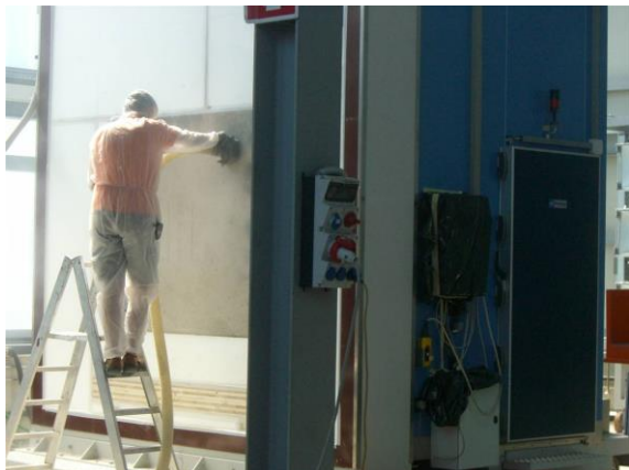
figure 82: Installation, © Elena Lucchi (Eurac)
