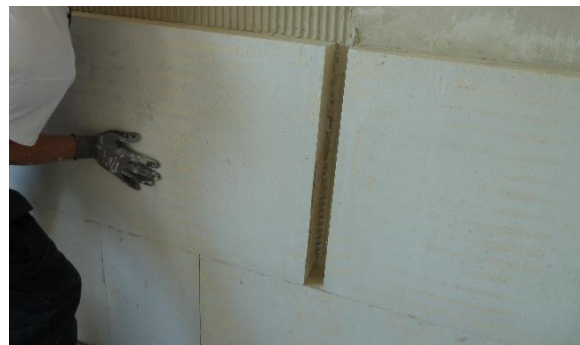
figure 11: Internally insulated gable wall, 80 mm of insulation (PUR-foam with thin calcium-silicate channels). Horizontal cross-section between external wall (insulated) and internal wall, including details at window (window sill insulated). © AAU
