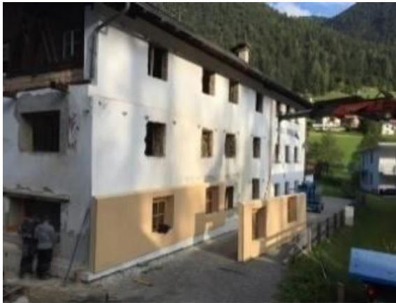
figure 156: Facade works, © Michael Flach
