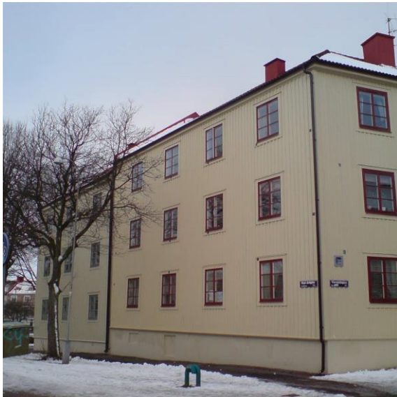
figure 114: Facade after intervention, © Pär Johansson
