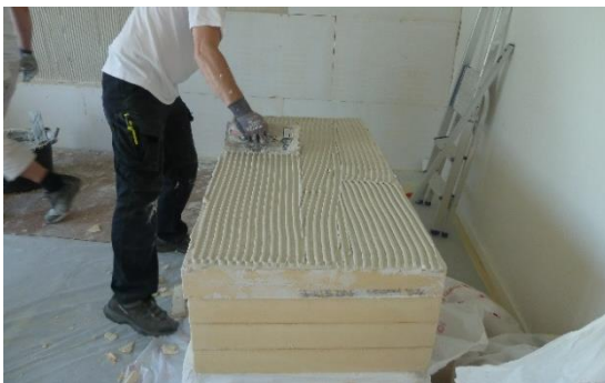
figure 12: Installation of internal insulation © AAU
