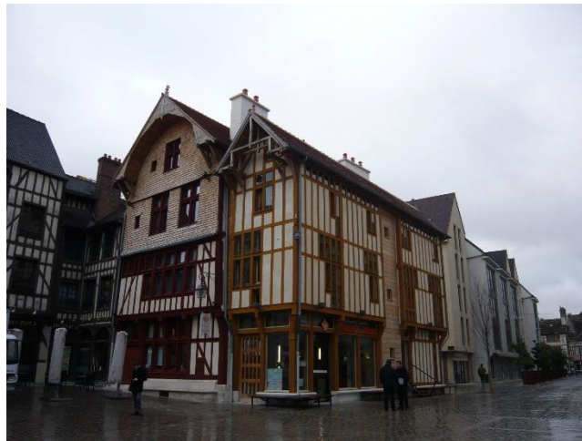
figure 159: Half-timbered house with hemp concrete infill, retrofitting (left part) and new construction (right part) in Troyes, tourism offices © Cerema
