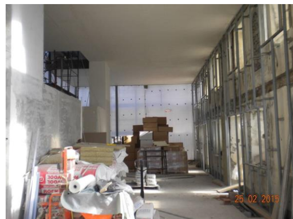
figure 54: During works: on the right metal profiles for fixing plasterboard © DeltaZero
