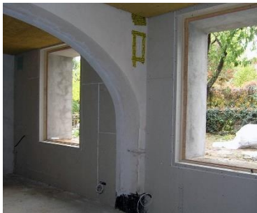
figure 43: Plaster Boards ©Eurac
