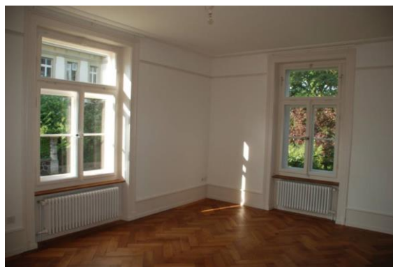
figure 77: Internal wall after intervention © M. Hutterli
