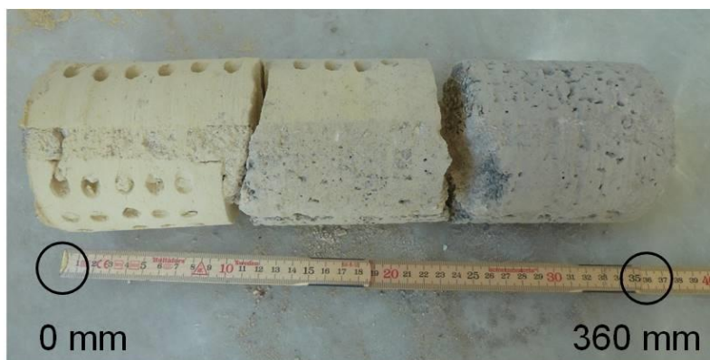
figure 9: Drill core of the wall structure. © AAU
