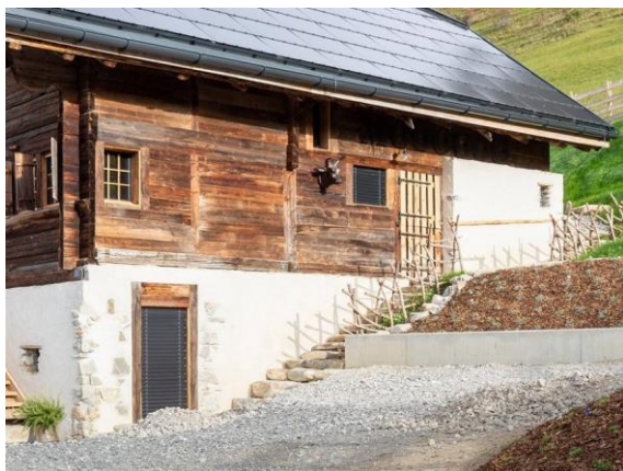
figure 144: New wood wall (side façade) © Daniel Baggenstos
