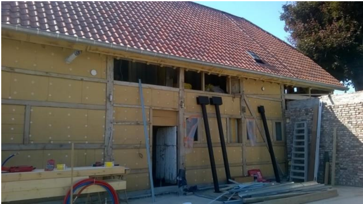
figure 180: Rear wall of the half timber-framed house in Alken during intervention
