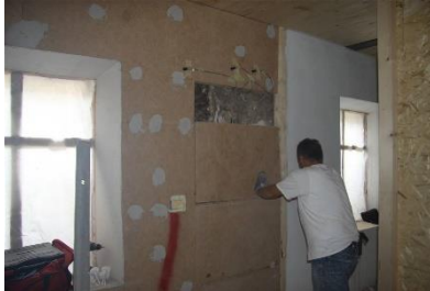
figure 23: Installation of wood fibre © Eurac
