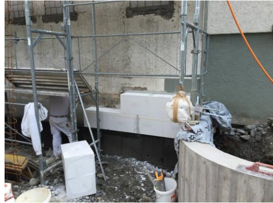
figure 121: Execution insulation, © City Chur
