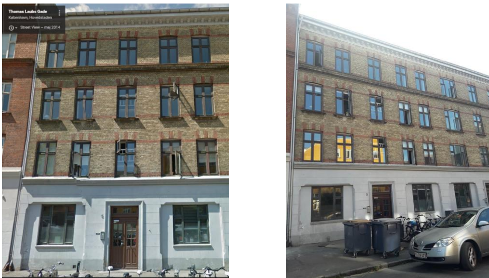
figure 8: Facade towards street. External wall in apartment at upper floor was renovated with internal insulation. © Google street view (left) and AAU (right)
