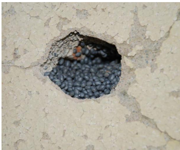
figure 74: Double-shell blowing system with Isofloc H2Wall © M. Hutterli
