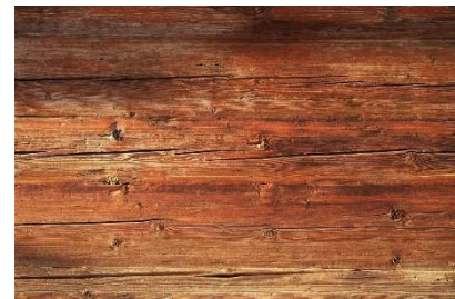
figure 68: old log wall © DI Alexander Rieser
