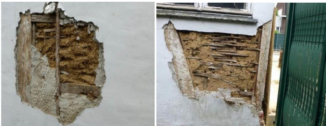
figure 177: Details of the original wall composition with wooden fence, visible wickerwork and loam (copyright Erfgoed en Visie bvba)
