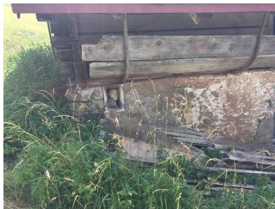
figure 145: Old wall before intervention © Gehret Design
