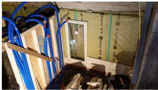
figure 71: Sheep wool with vapour control layer, ©Benjamin Schaller
