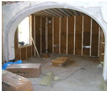
figure 44: Internal insulation in the sleeping room: wood fibre ©Eurac
