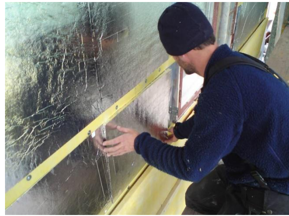
figure 113: Mounting of vacuum insulation panels, © Pär Johansson
