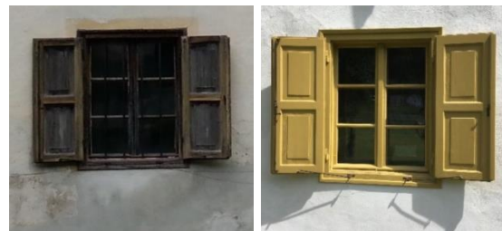
Knablhof (box-type window) – before and after renovation.
