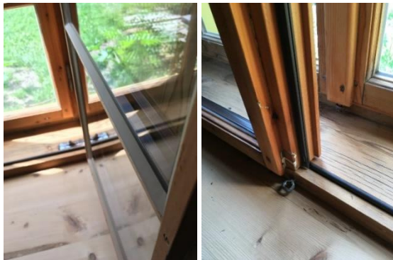
Knablhof (box-type window) – details after renovation
