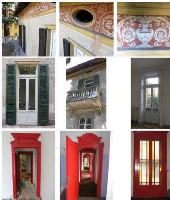
Villa Castelli, Bellani, Italy pre intervention
