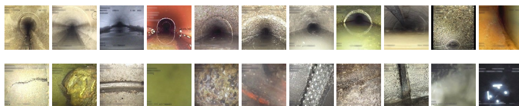
Figure 2. Examples from the Sewer-ML database. First row from left to right: 0%, 10%, 20%, 30%, 40%, 50%, 60%, 70%, 80%, 90% and 100% water level percentages. Second row shows examples where the water level is ambiguous.
