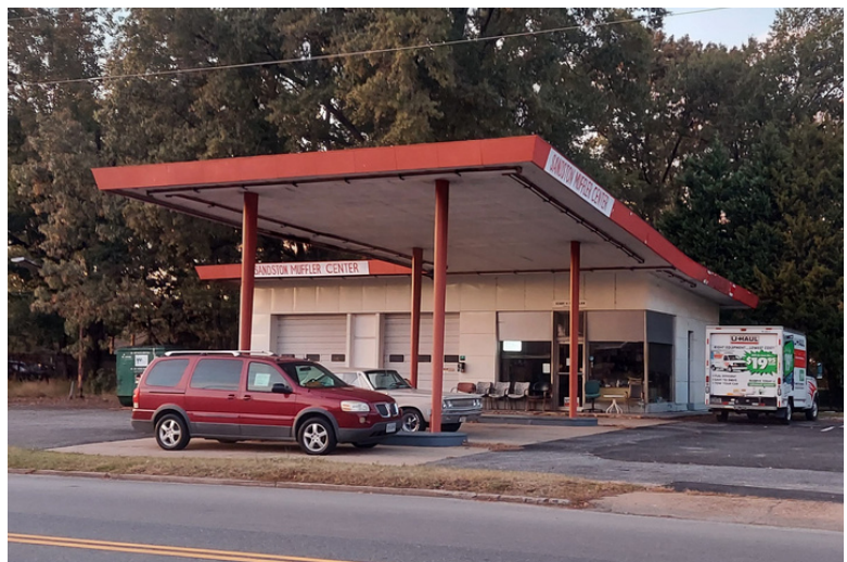
Figure 1: A gas station located on the western end of Williamsburg Road.
