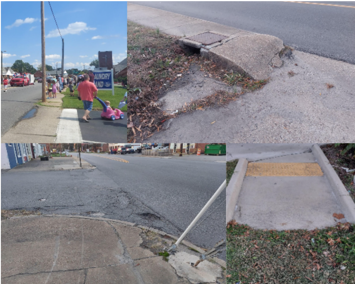
Figure 4: Examples of deteriorated sidewalks with leftover pooling water from a previous rain, uneven walkways, broken asphalt and concrete, and random discontinuation of sidewalks.
